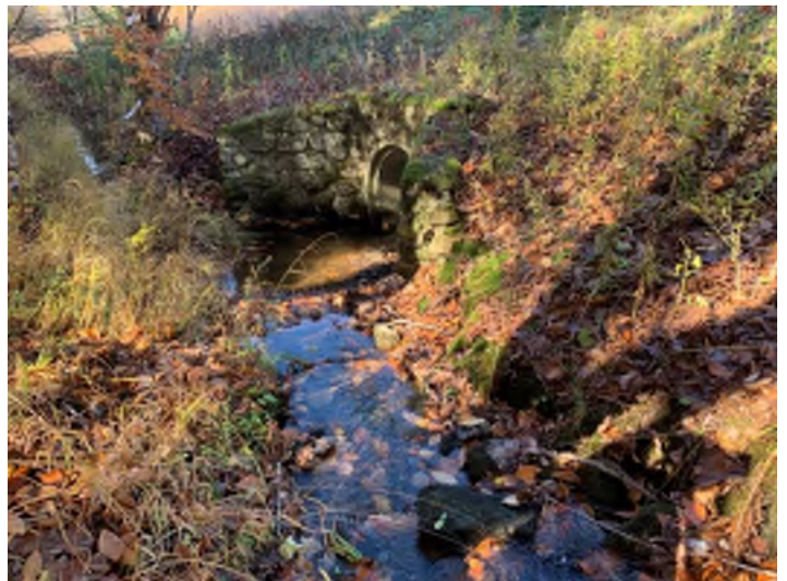
Photo 24. An image of the inlet at Crossing 6 SB 1287+40.
