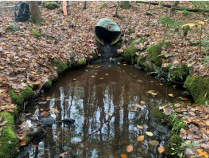
Photo 9. A scour pool is located at the perched outlet of Crossing 4 NB 1199+75.
