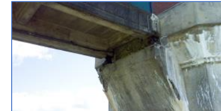
High resolution inspection photo of a structure at Murphy Dam.
