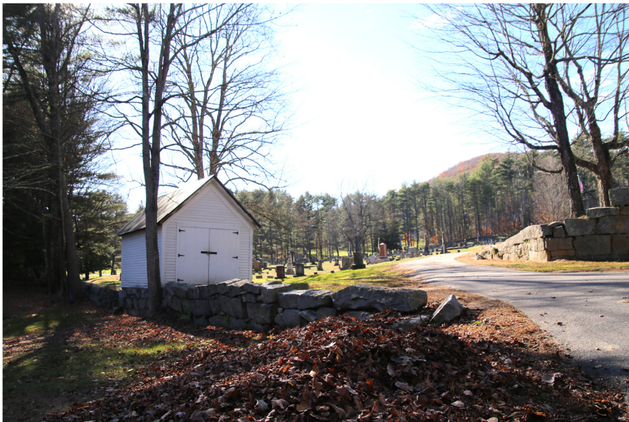
The hearse house, built in about the 1890s, was designed for a horse-drawn vehicle. The granite receiving tomb was constructed in 1859 by stone mason Alfred Seaver of West Swanzey.
