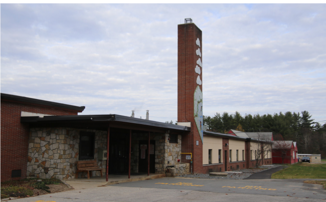
The red brick building retains its original stone veneer front with recessed entry and tall rectangular brick chimney. The many large windows were filled in for energy efficiency in 2016.
