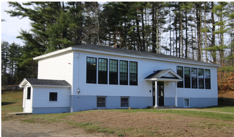
The building looks unchanged even though it had indeed changed from the original. After a tree fell on it in 2013, it was restored with a new roof, siding, doors, and windows that replicate the originals.
