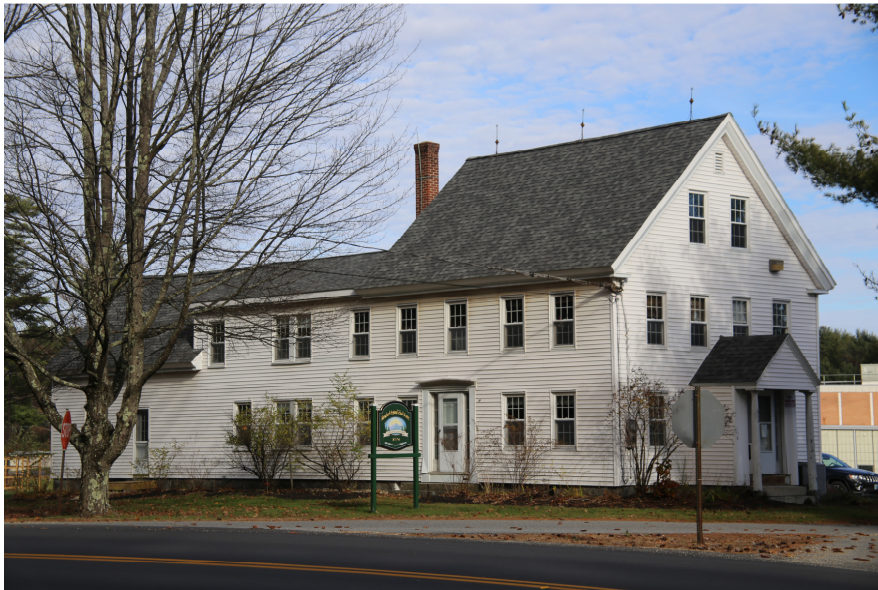
The original form of the farmhouse and the Greek Revival style front entrance are unchanged though the siding and windows are all new. Some of the farm outbuildings can be seen among the high school shops.
