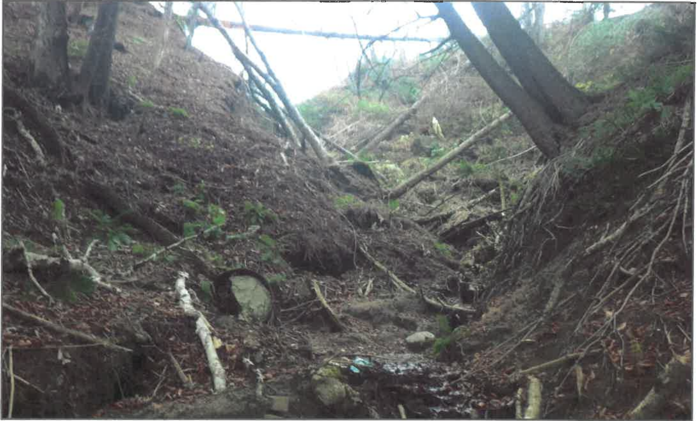
Photo 7: Looking North from bottom of failure, location of groundwater 'daylight'
