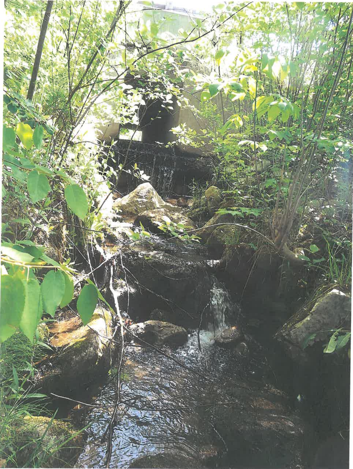
Impact Area D (west of US 3)- permanent bank & Impact Area C (west of US 3)- permanent channel
