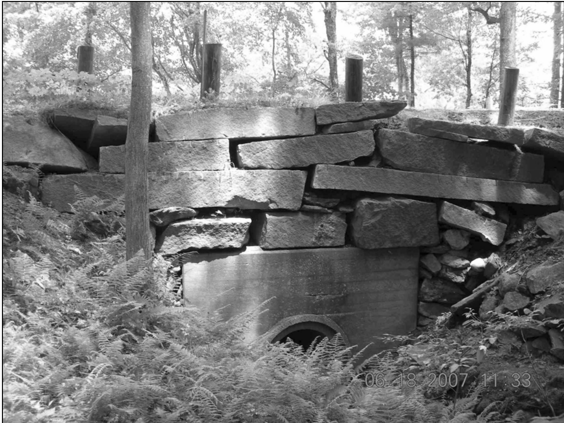
Photo No. 20: Culvert TRO0344 (Troy)
