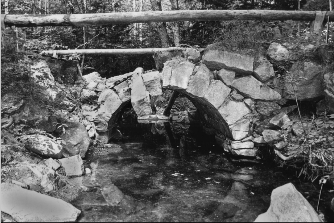
Photo No. 15: Culvert TEM0002 (Temple)
