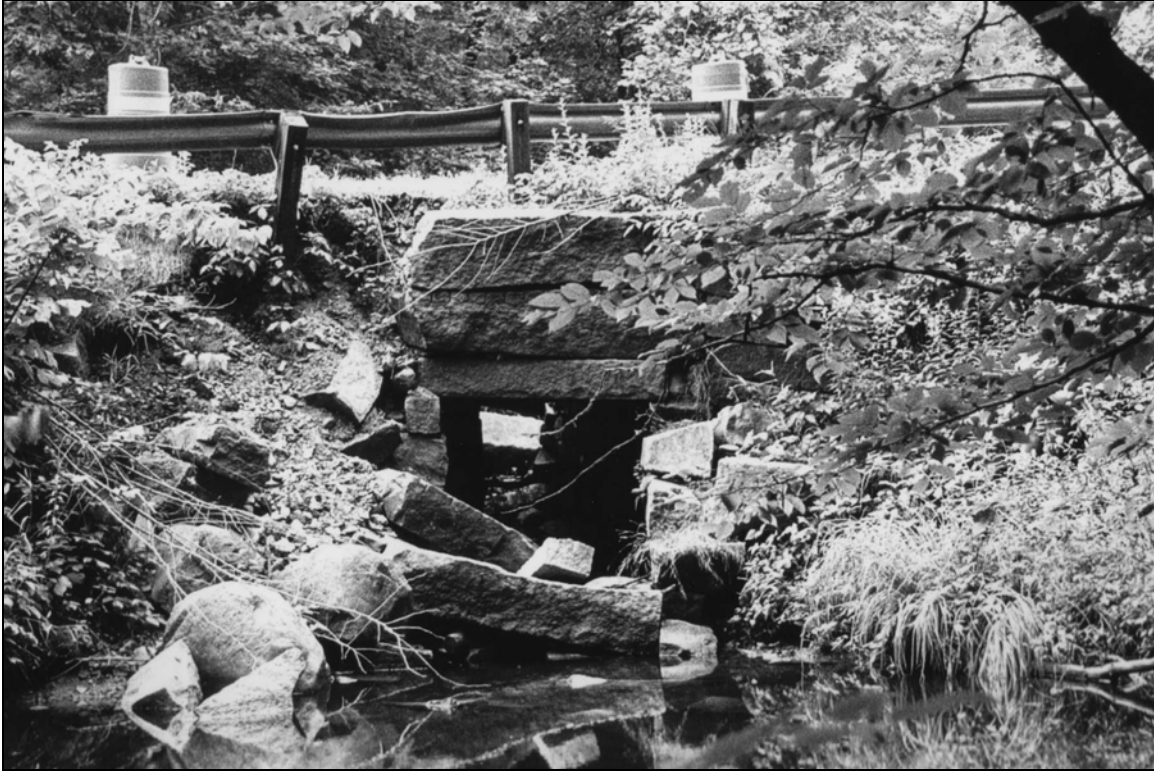
Photo No. 14: Culvert HIL0144 (Hillsborough)
