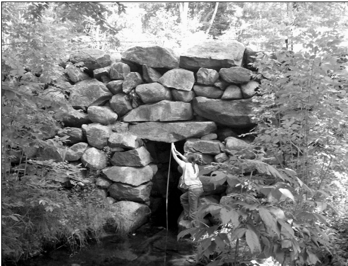
Photo No. 3: Culvert TUF0007 (Tuftonboro)
