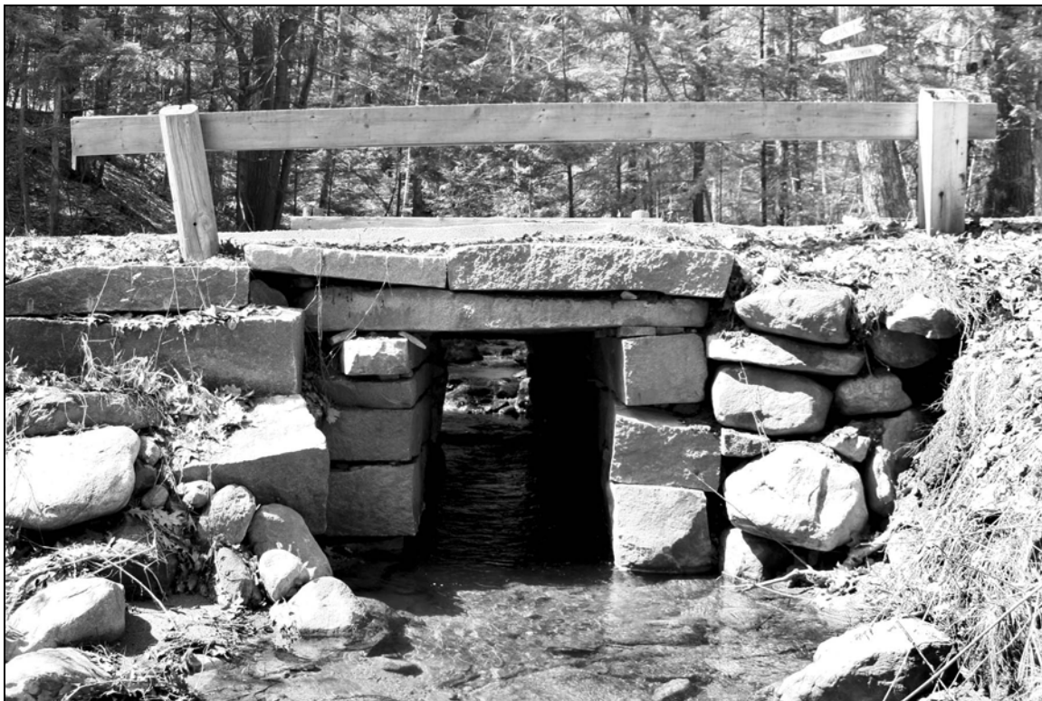
Photo No. 8: Culvert MAR0015 (Marlborough)
