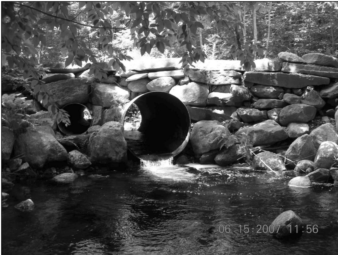
Photo No. 17: Culvert SWA0019 (Swanzy)
