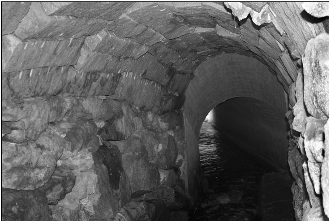
Photo No. 16: Culvert LIT0010 (Litchfield)
