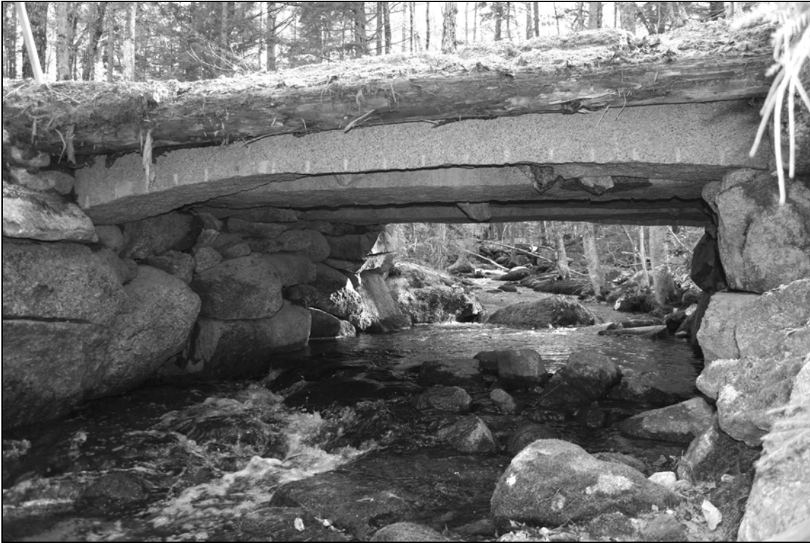
Photo No. 1: Culvert HIL0019 (Hillsborough)
