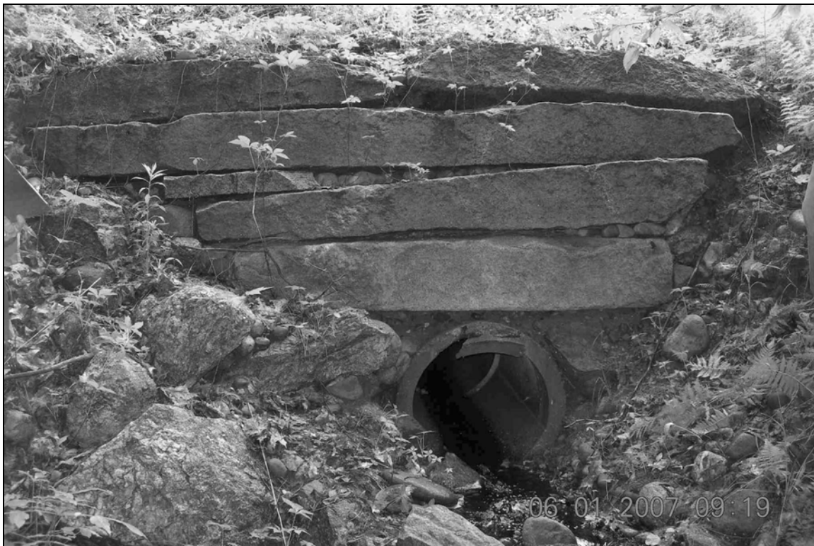
Photo No. 18: Culvert PEM0040 (Pembroke)
