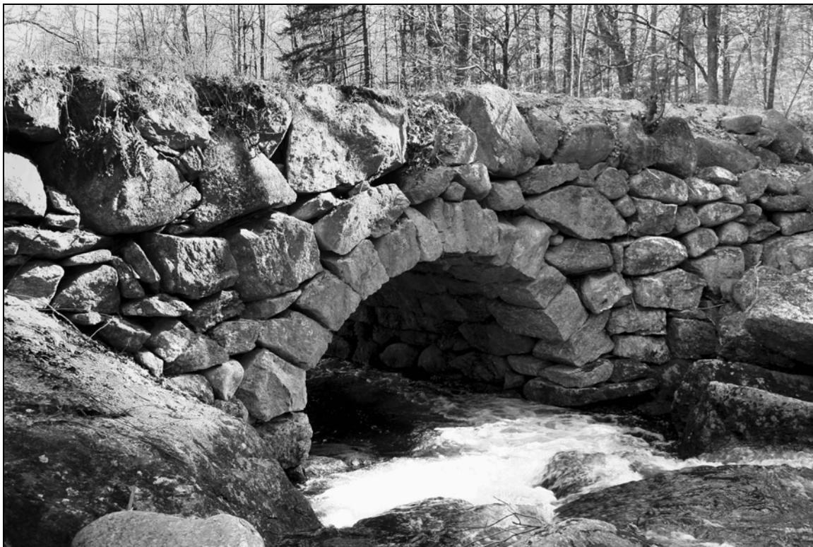
Photo No. 11: Culvert HIL0022 (Hillsborough)
