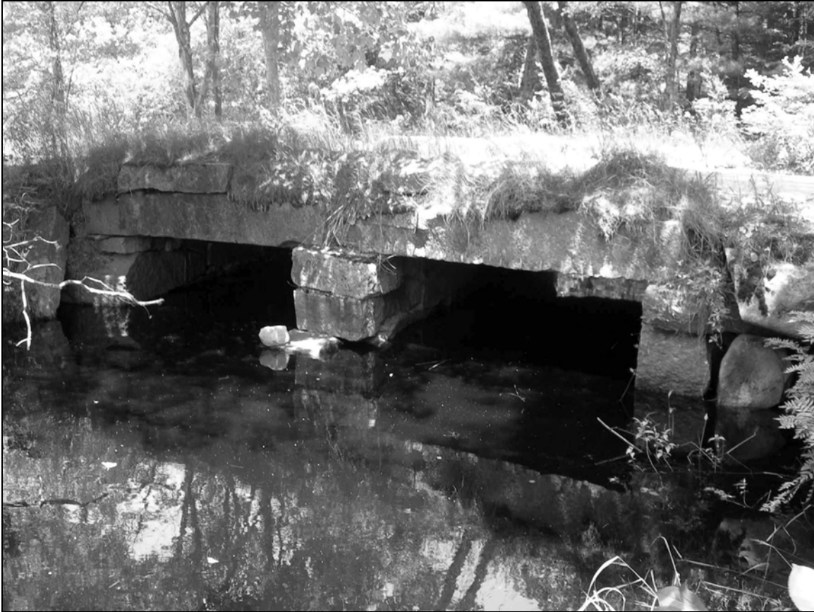
Photo No. 4: Culvert FIT0017 (Fitzwilliam)
