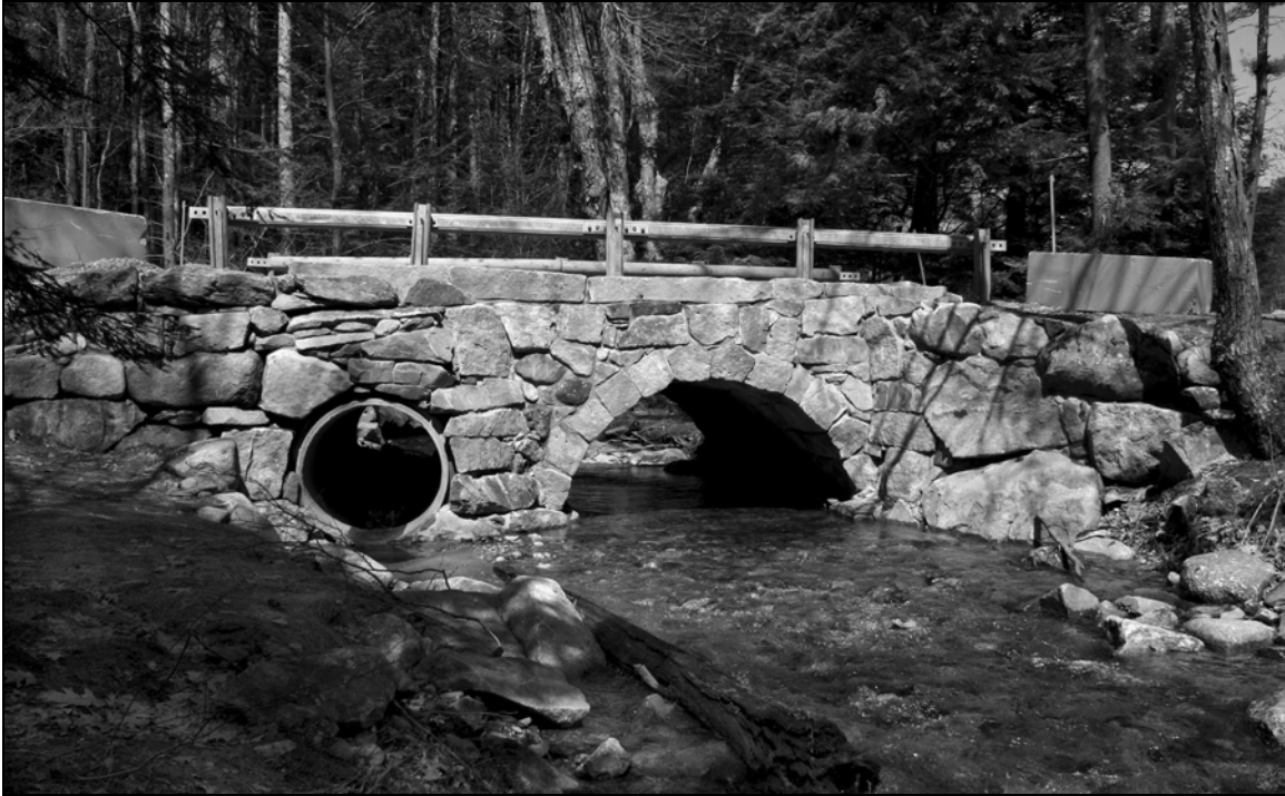
Photo No. 24: Culvert TEM0002 (Temple)
