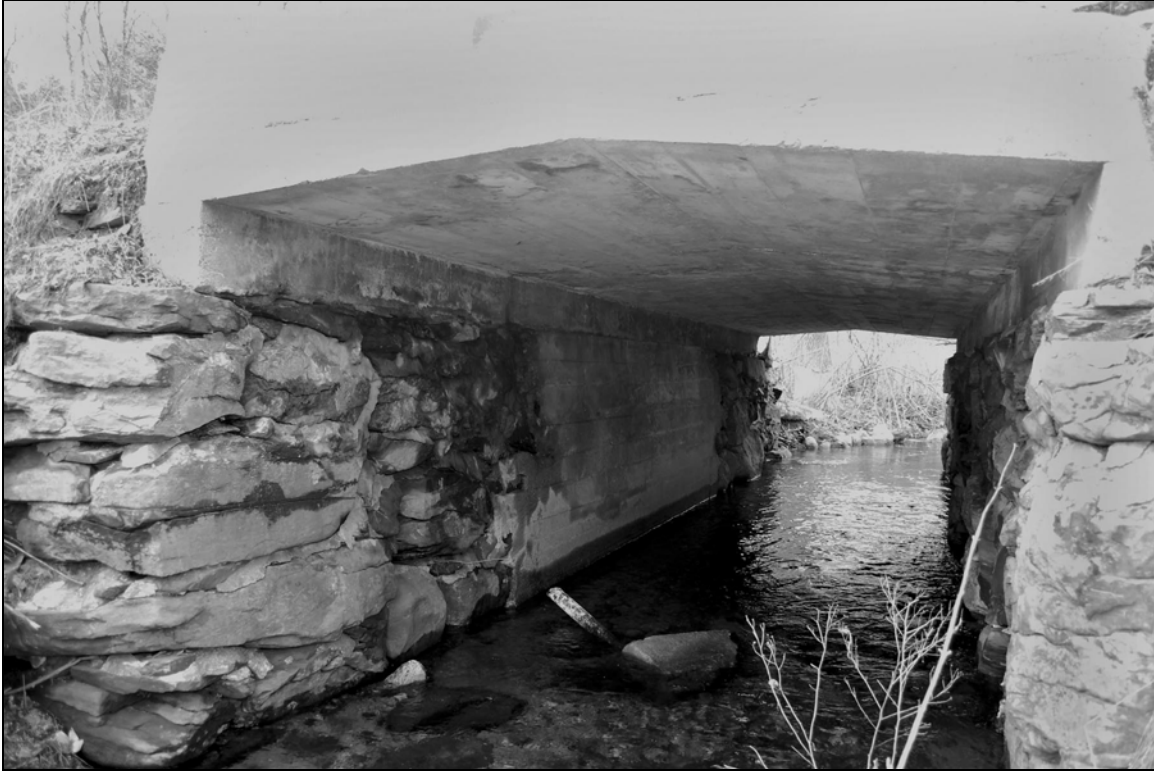
Photo No. 22: Culvert LON0112 (Londonderry)
