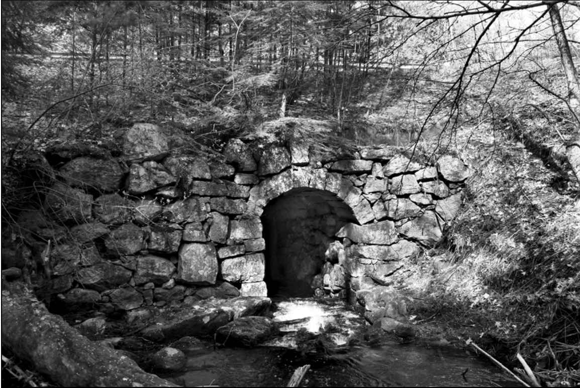
Photo No. 10: Culvert LIT0010 (Litchfield)
