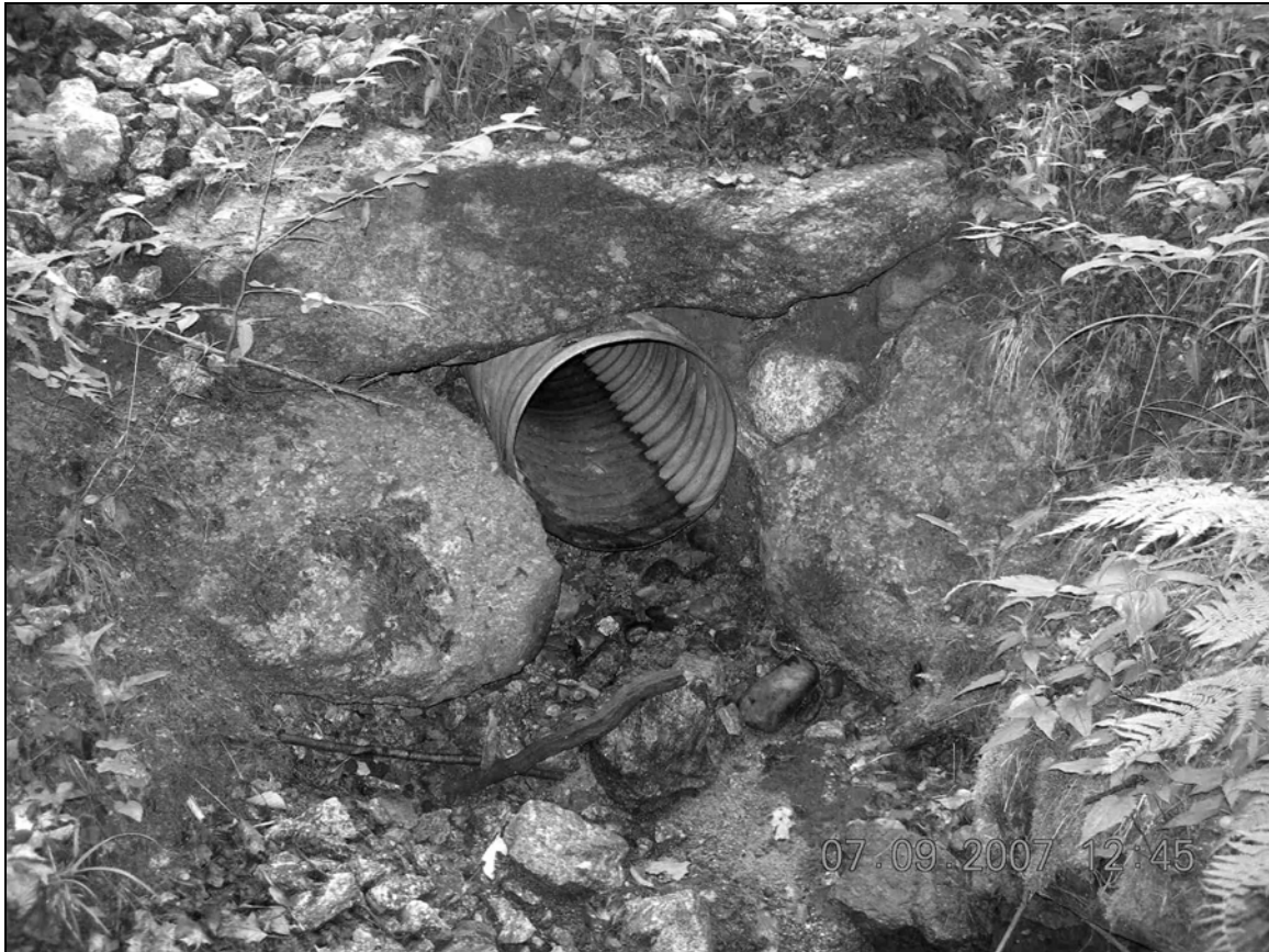
Photo No. 19: Culvert NBR0004 (Newbury)
