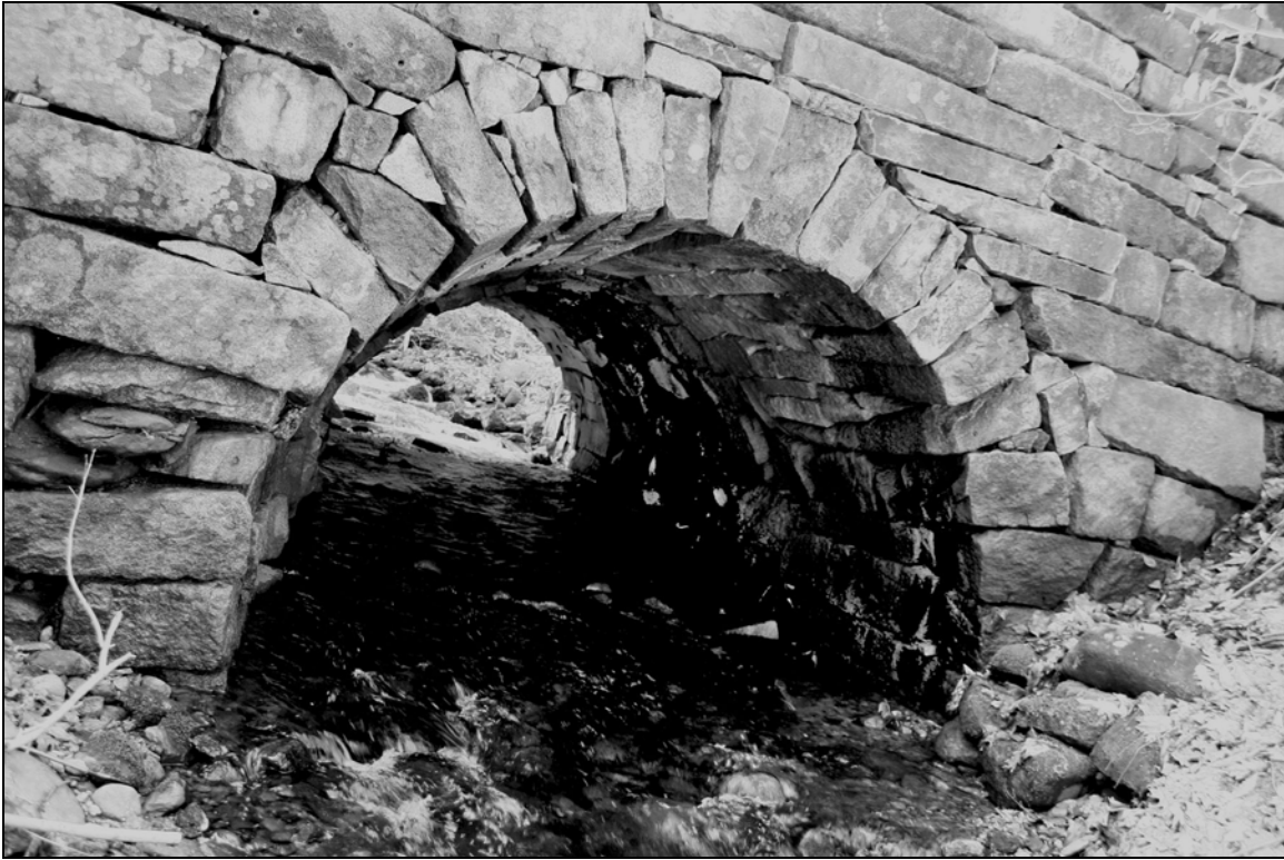
Photo No. 12: Culvert WIL0006 (Wilton)
