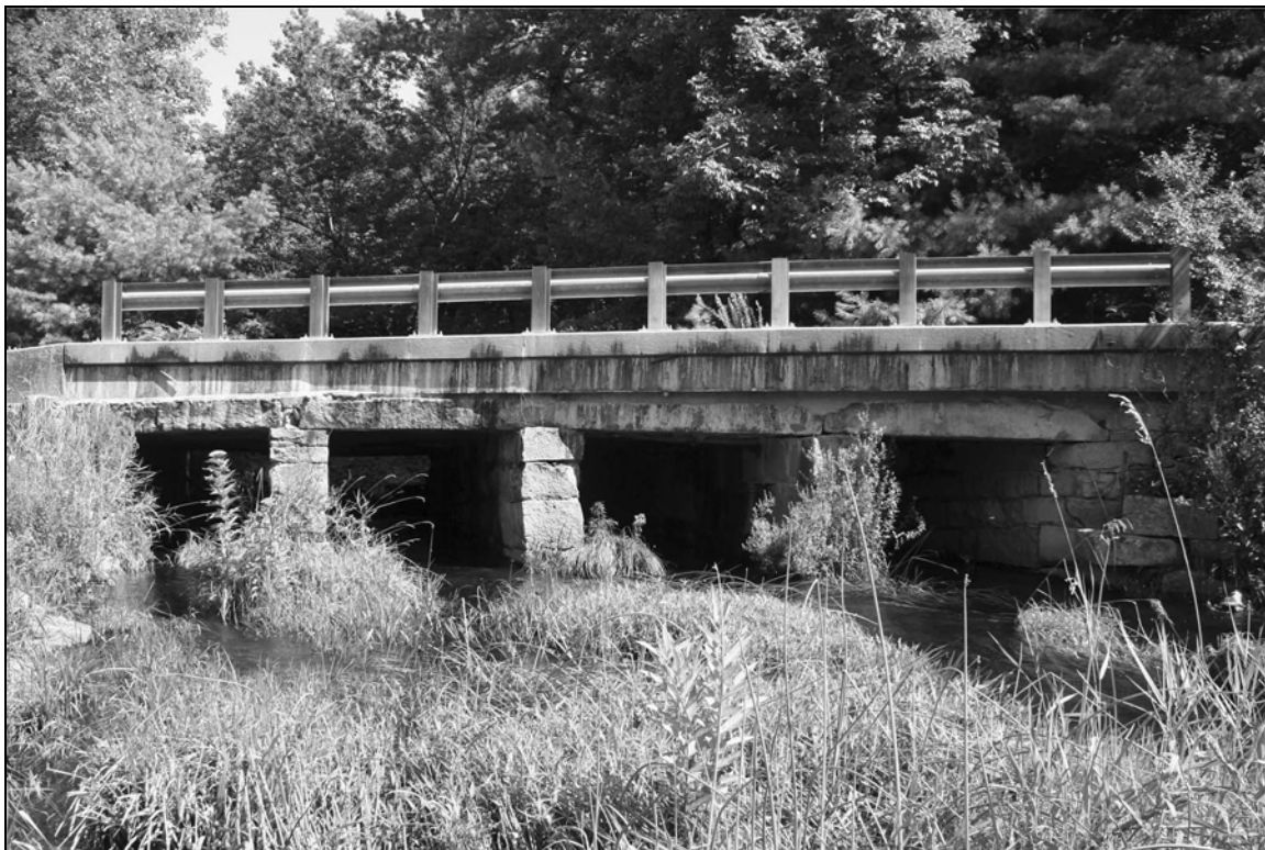
Photo No. 6: Amherst Bridge 159/105 (Amherst)
