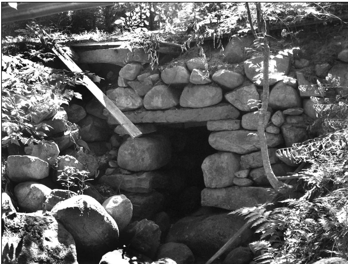
Photo No. 7: Culvert WOL0026 (Wolfeboro)
