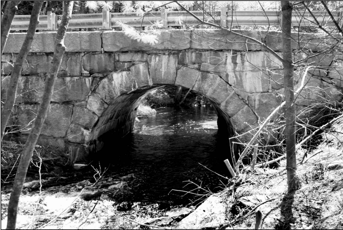
Photo No. 9: Culvert JAF0464 (Jaffrey)
