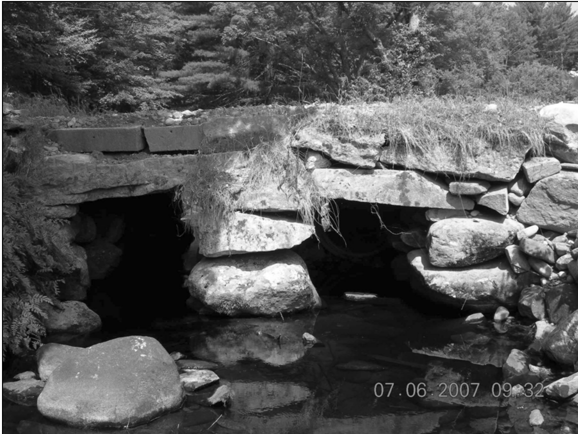
Photo No. 5: Culvert CNT0007 (Canterbury)
