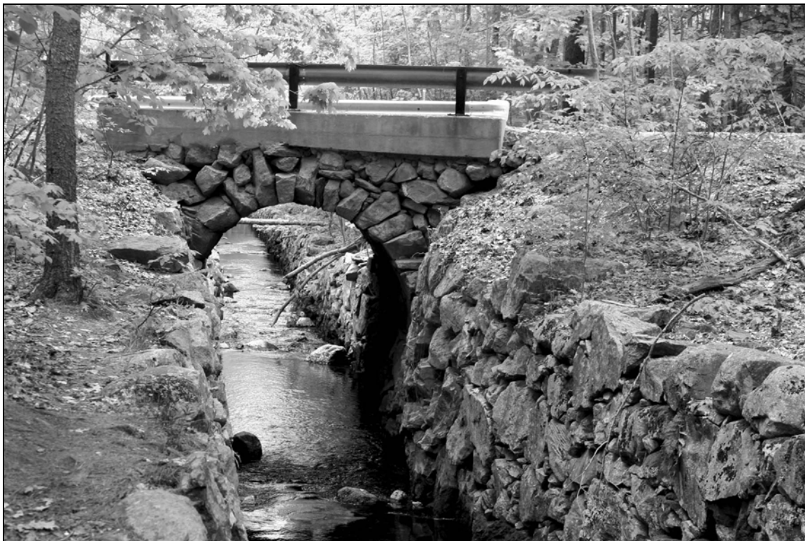
Photo No. 21: Culvert WAK0010 (Wakefield)
