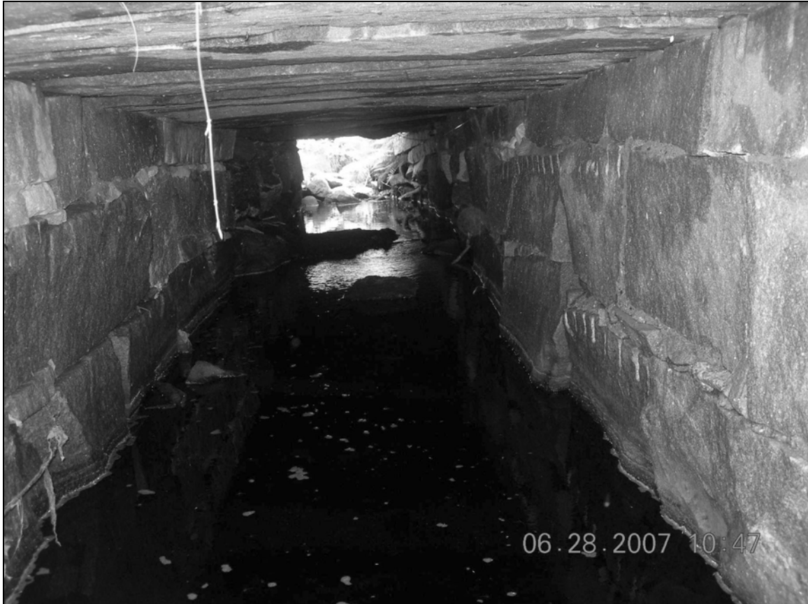
Photo No. 23: Culvert FIT0015 (Fitzwilliam)
