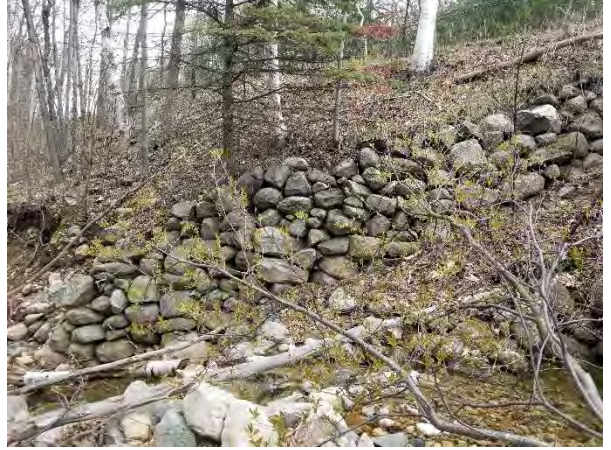
Photo 8: Rock wall along east of the culvert outlet
