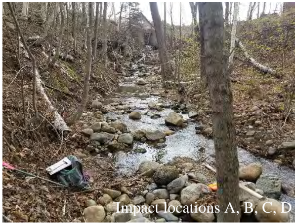
Photo 9: Northern end of the study area looking upstream towards the culvert outlet
