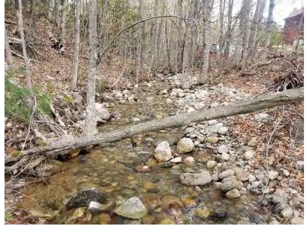
Photo 2: Culvert inlet facing upstream
