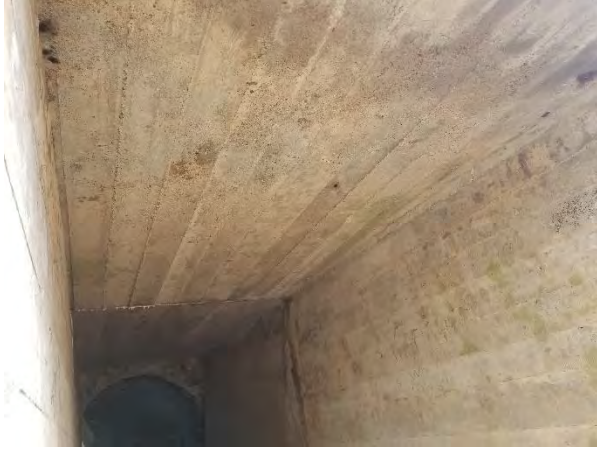
Photo 7: Inside box culvert portion of the crossing
