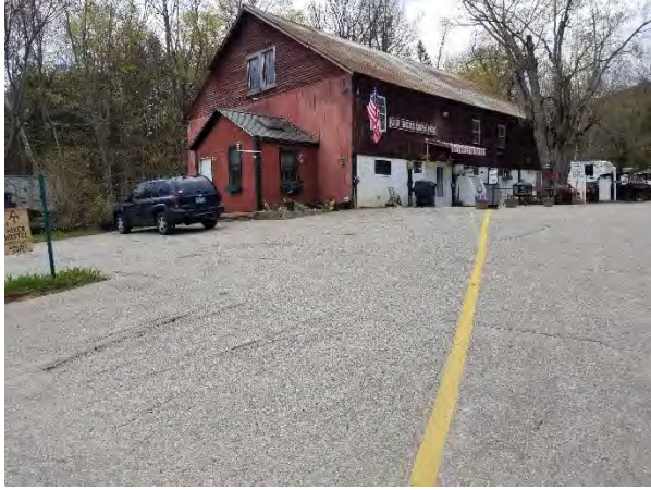
Photo 13: Adjoining property to the southwest of the crossing. White Birches Campground.
