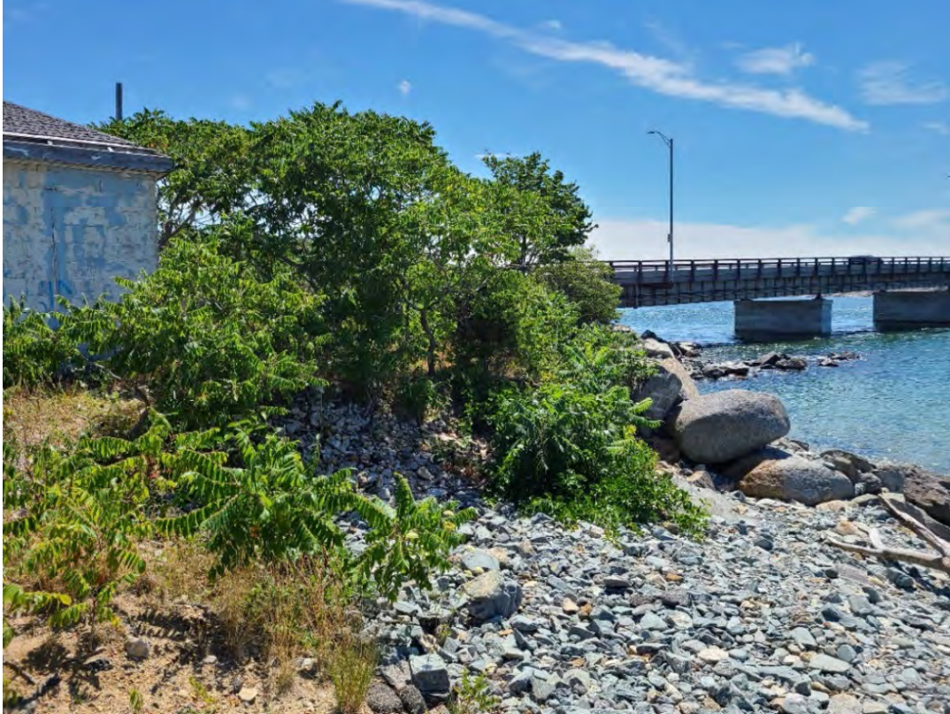
Northwest Quadrant: Looking southeast at bridge in TBZ showing shrub vegetation
