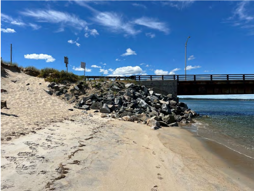
Southeast Quadrant: Looking west at bridge in TBZ and Intertidal area
