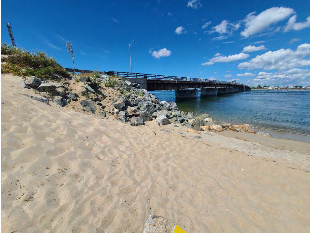
Southeast Quadrant: Looking northwest at bridge in TBZ
