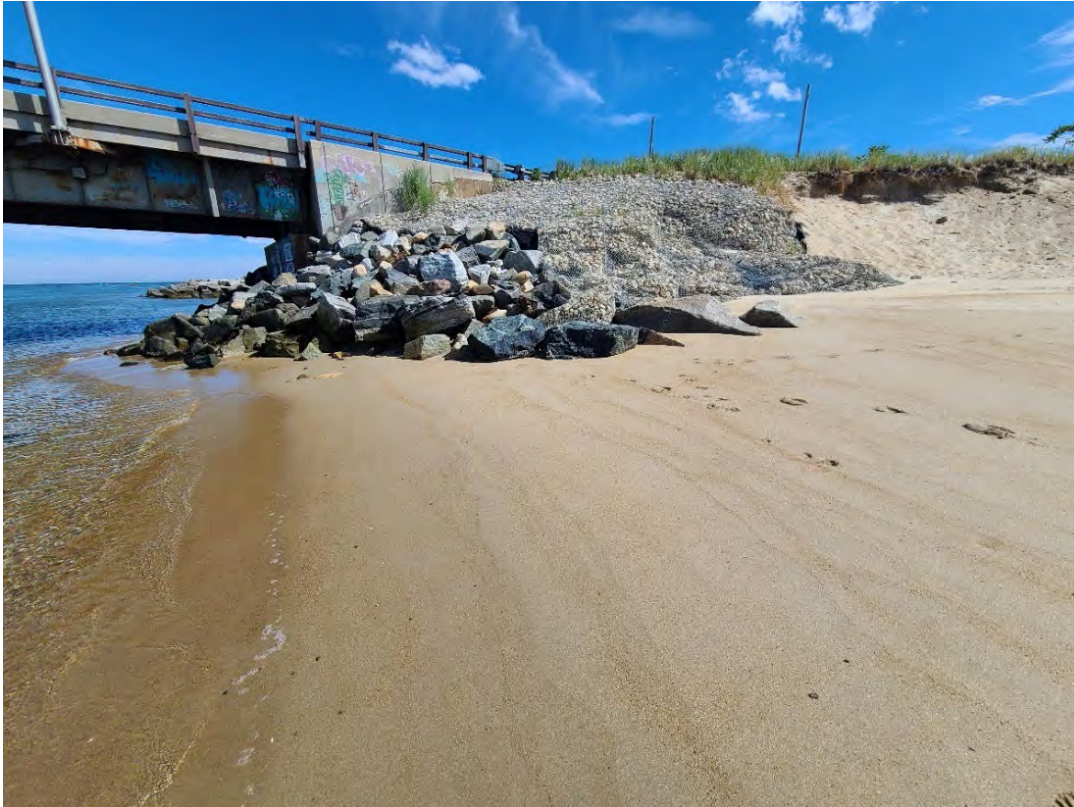
Southwest Quadrant: Looking east at bridge in TBZ and intertidal area
