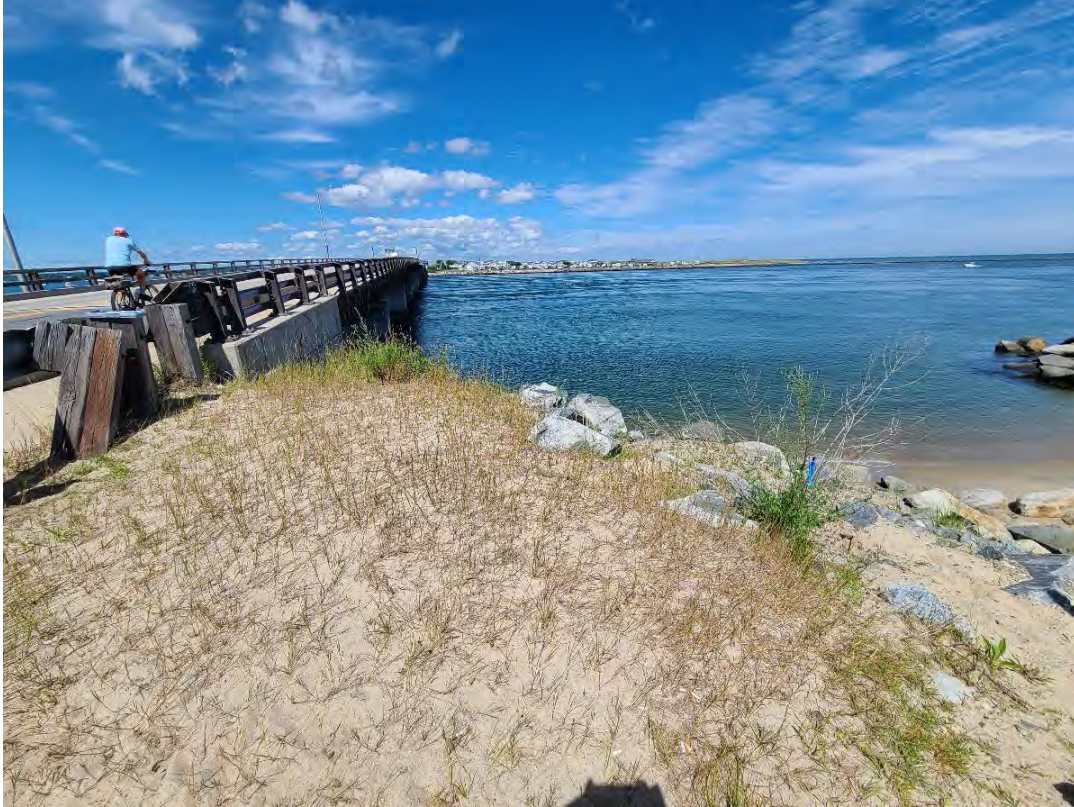
Southeast Quadrant: Looking north along east side of bridge in TBZ
