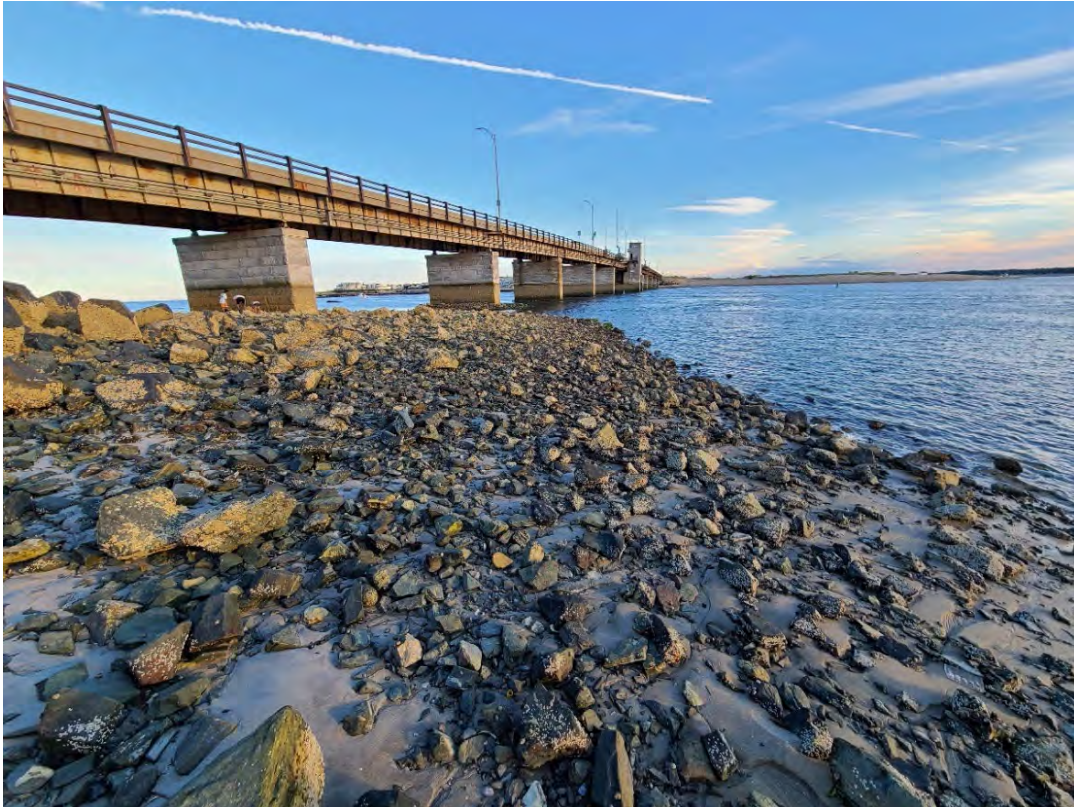
Northwest Quadrant: Looking southeast at bridge in intertidal area
