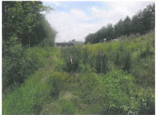
Photo 22. Wetland M-5 is a constructed stormwater treatment wetland on the side of I-93.
