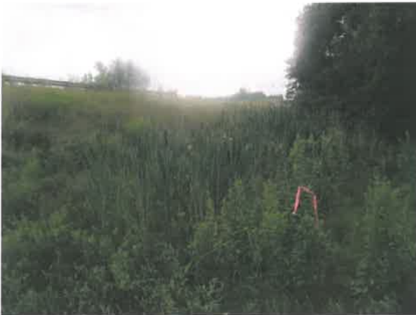
Photo 21. Wetland M-4 is a constructed stormwater treatment wetland on the side of I-93.
