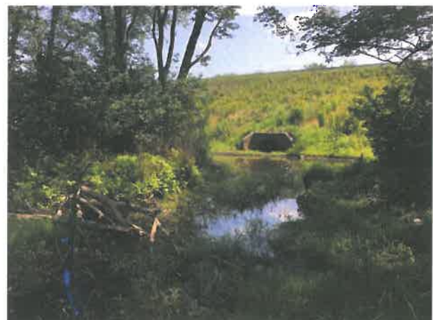
Photo 54. Stream S-S4 traverses wetland S20.
