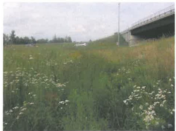
Photo 24. Wetland M-7 is a constructed stormwater treatment wetland in the highway median.
