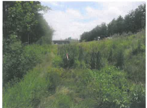
Photo 22. Wetland M-5 is a constructed stormwater treatment wetland on the side of I-93.
