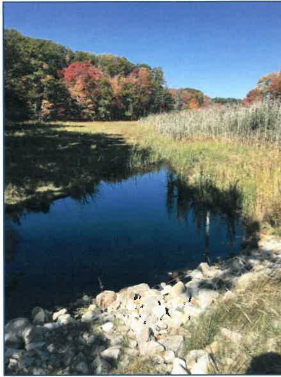
Photo 13- View west along Wetland area A3 (estuarine intertidal marsh with common reed), taken standing atop Route 1A. Riprap and twin 36" HDPE culvert inverts clearly visible in foreground.
