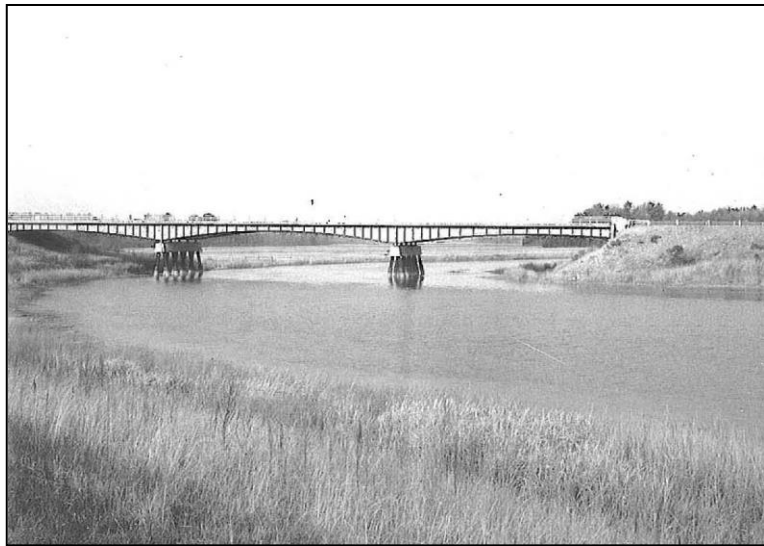
Figure 10. Squamscott River Bridge (Bridge No. 106/100) between Exeter and Stratham. Source: NHDOT Bridge Card.
