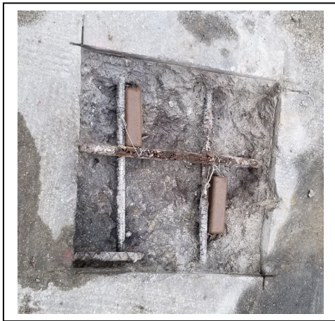
Discrete Anodes (Partial-depth Deck Repair)
