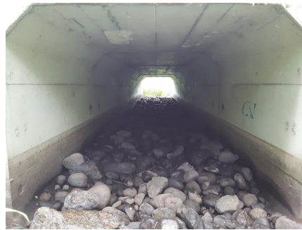
An embedded culvert in Londonderry, NH, that is hyporheic (movement of stream water into the subsurface).
