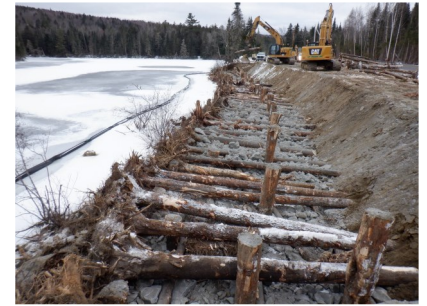
Stacked members of ELJ installation
