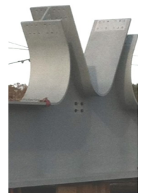
A gusset-less connection from Memorial Bridge
