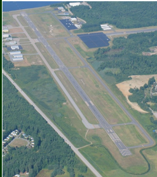
In this aerial view of Laconia Airport, the white runway paint is heavily stained and appears yellow.
