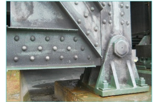
Typical Truss Bearing
