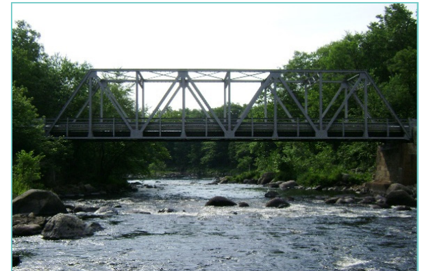
Ramsdell Road Bridge, Henniker, NH
