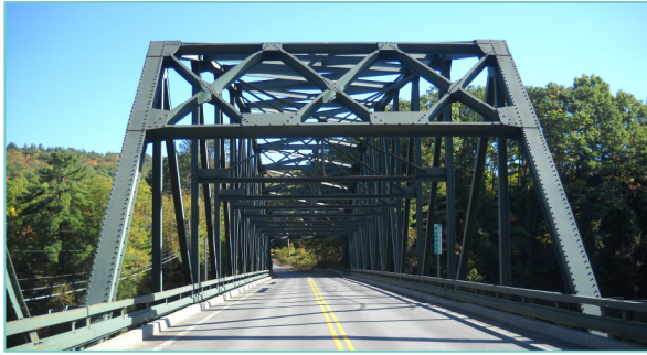
Barnet Road Bridge, Monroe, NH
