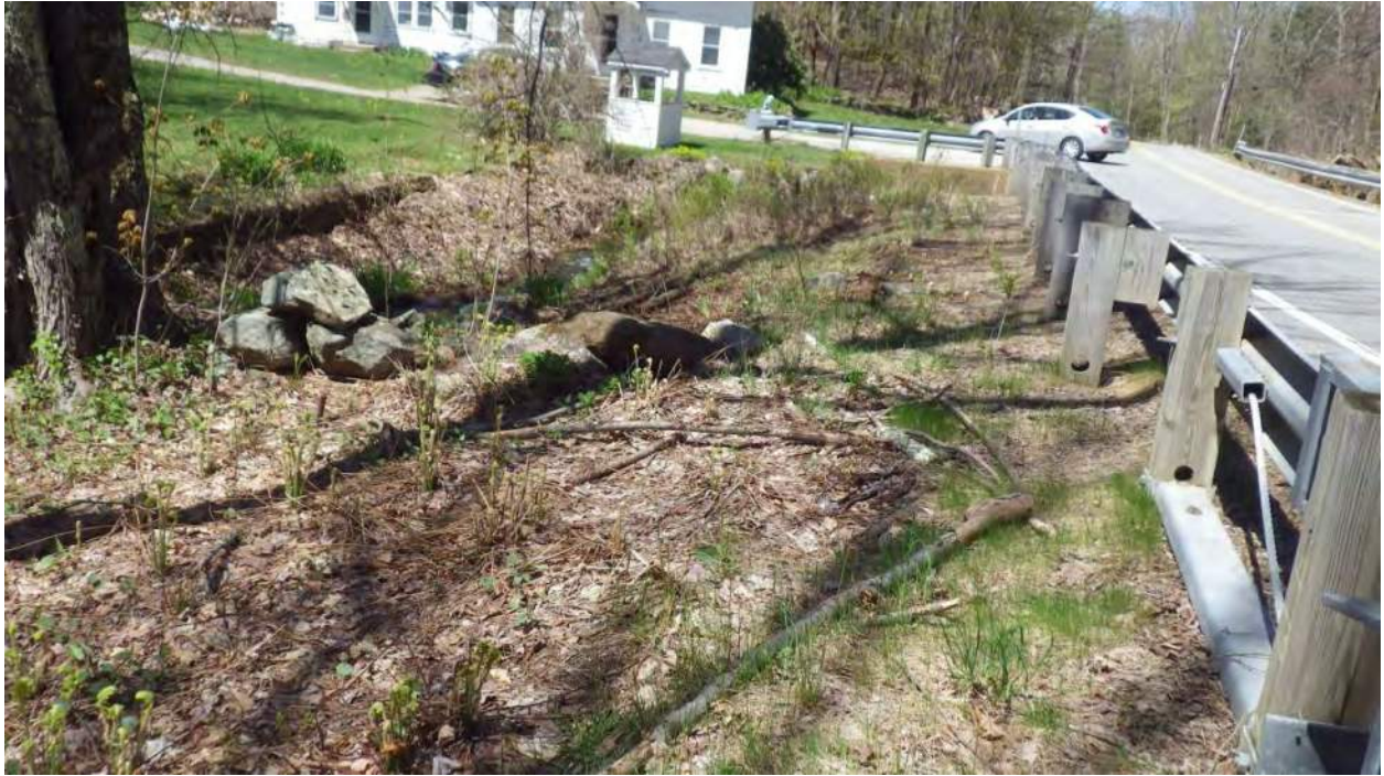
Photo 1: Inlet looking North down NH Route 107
