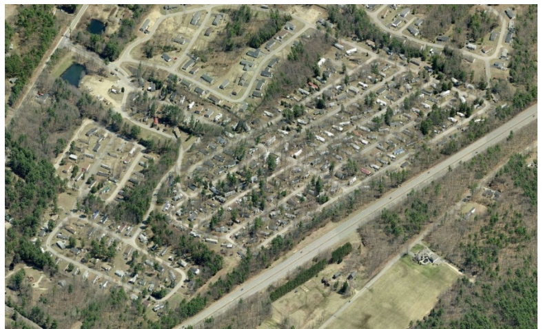
Dense Residential Neighborhood near a Tier 1 Highway
