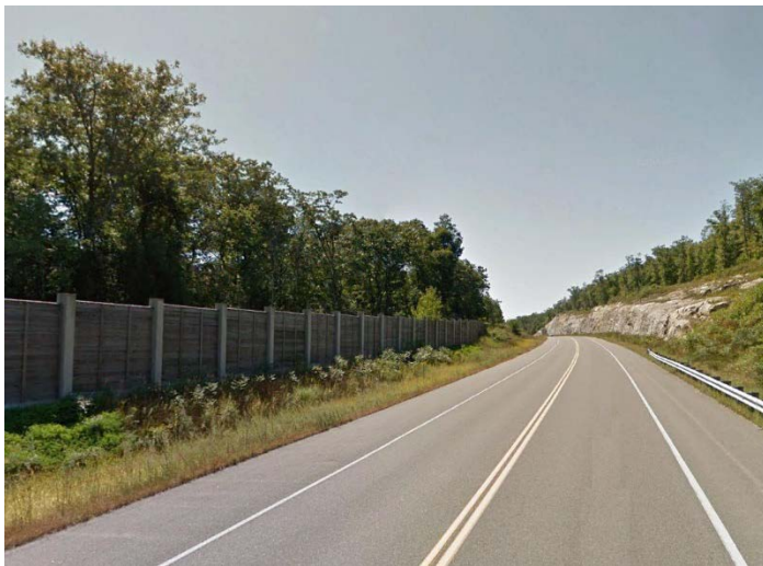
Typical Highway Noise Barrier
