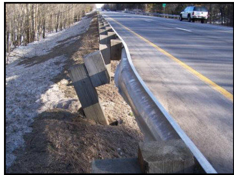
Fig 9 and 10: Damage on I-93 at MM 63.4 northbound, along the high speed lane in March 2011
