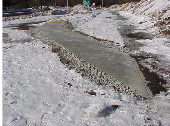
Ramp uncovered on February 26, 2003
