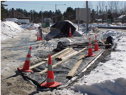
During curing, February 20, 2003 North Ramp, Looking South
