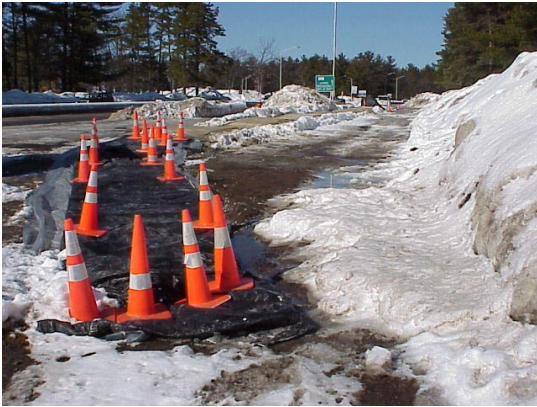
During curing, February 20, 2003 South Ramp, Looking North
