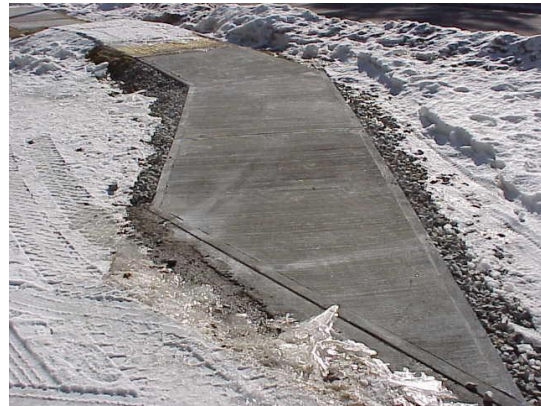
Ramp uncovered on February 26, 2003
