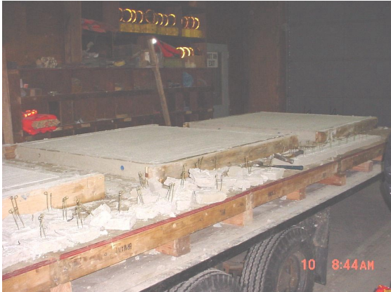
Concrete panel fabrication in the Bridge Maintenance Bureau shop
