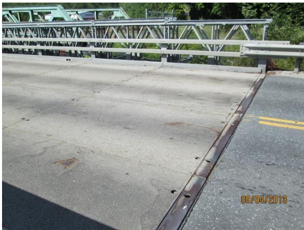
Figure 1. PolyCarb Flexogrid delamination on the Acrow temporary bridge deck panels
