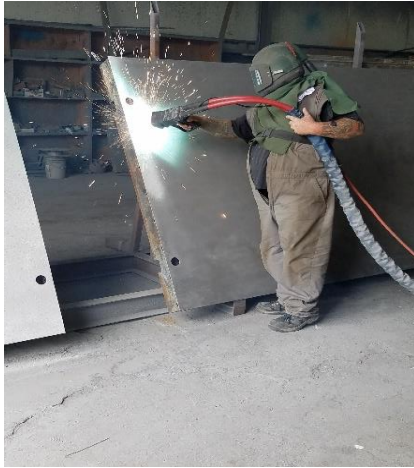
TSC Application In-Process
