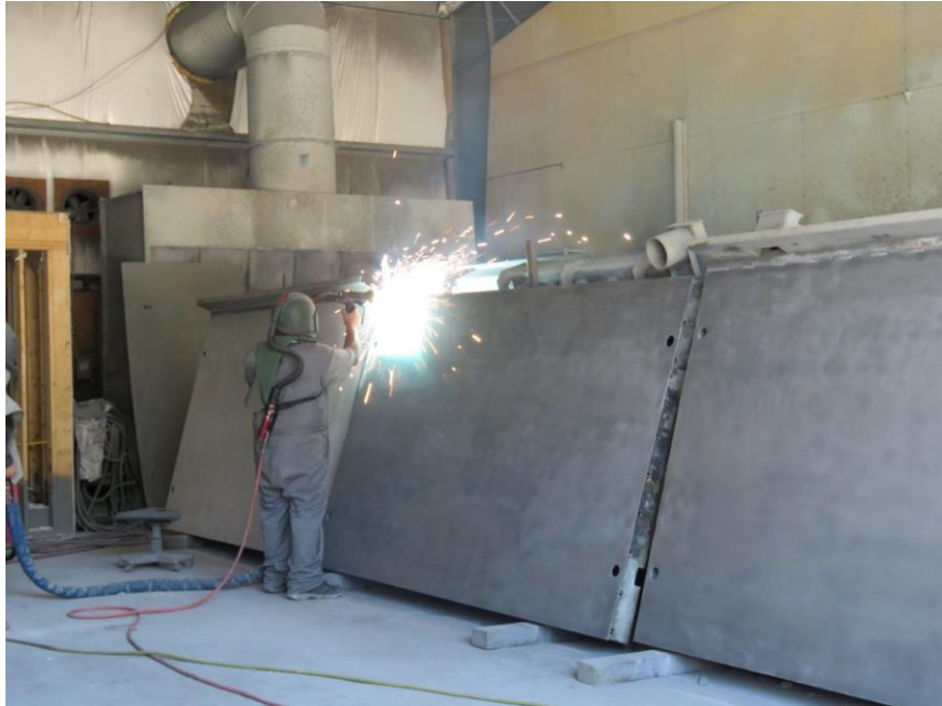
Figure 1: Thermal spray top coat being applied to bridge deck panel.
