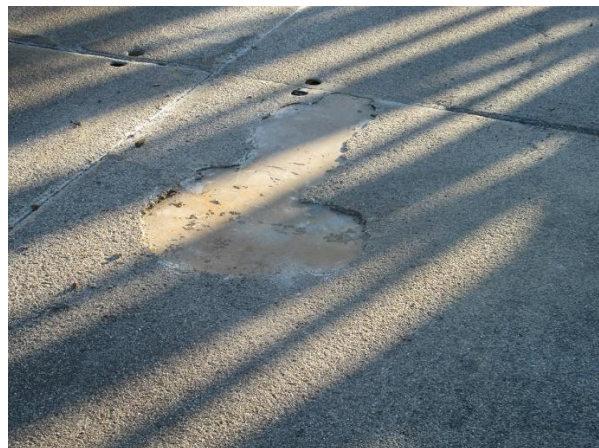
Figure 1. PolyCarb Flexogrid delamination on the Acrow temporary bridge deck panels
