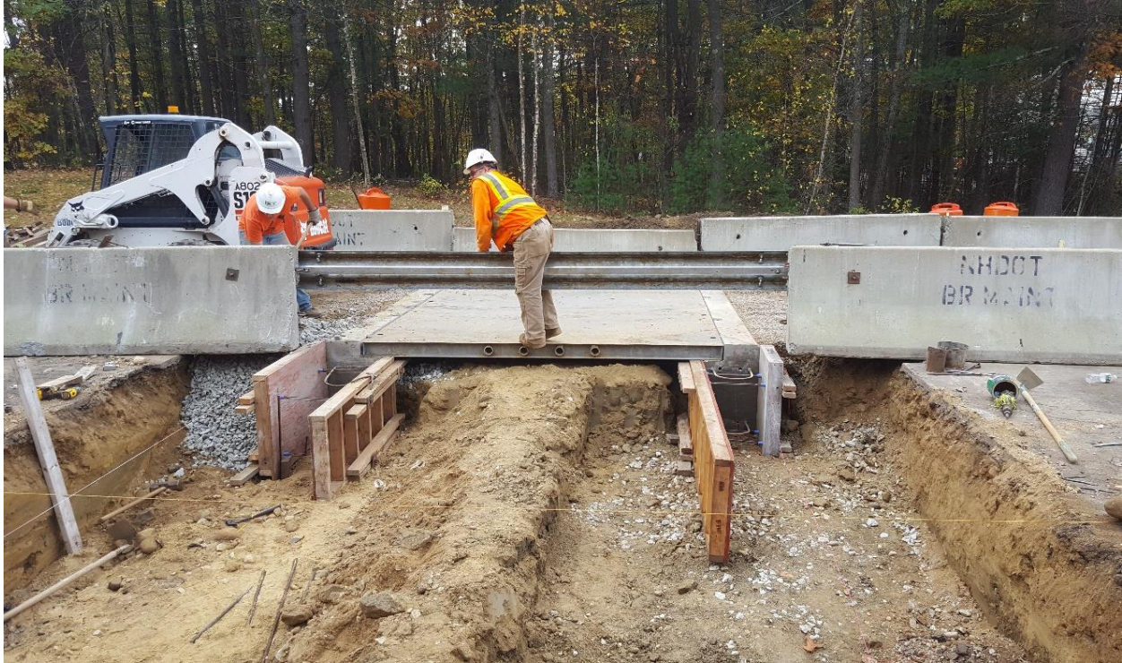
Figure 3. The panel installation at the NHDOT maintenance shed in Newfield, NH
