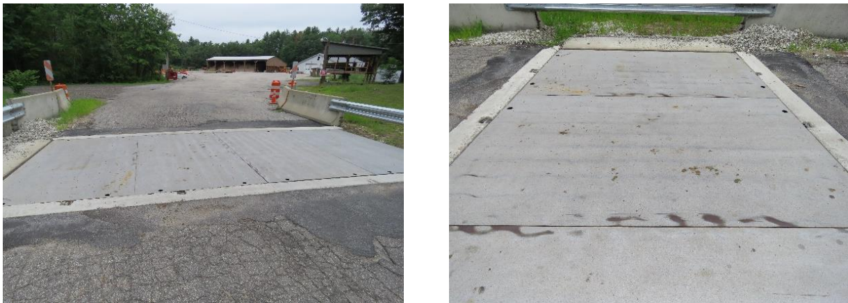
Figure 4. Post-trafficking images of Acrow bridge panels with Thermion SafTrax TH604 Metallized Coating
