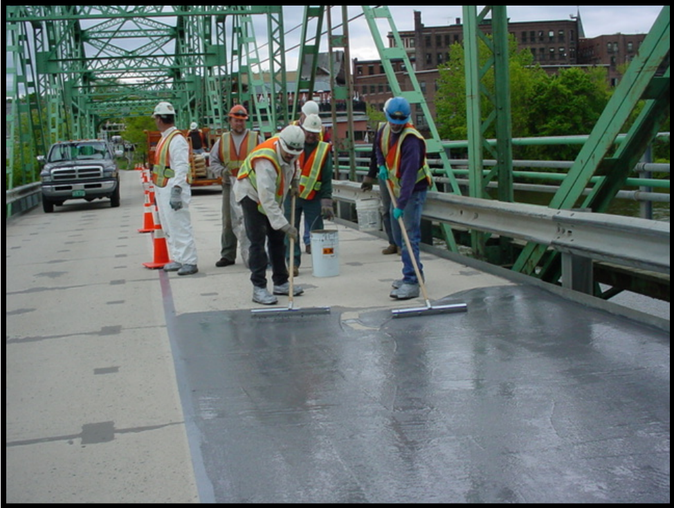
Figure 5 – NHDOT Bridge Maintenance installing Stirling Lloyd product
