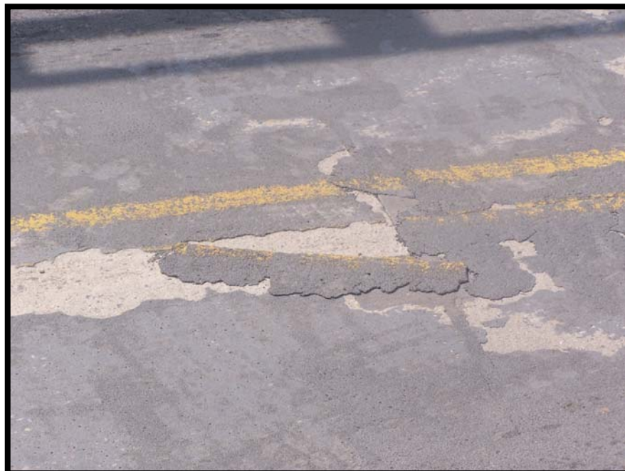
Figure 12 – Separated pieces of Stirling Lloyd
