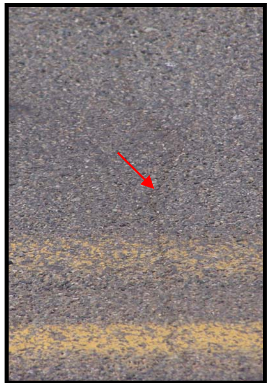
Figure 10 – Flexogrid cracking
