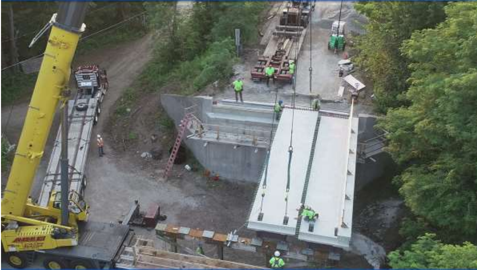
Prefabricated Bridge Units (PBU's) & Ultra-High Performance Concrete (UHPC)
