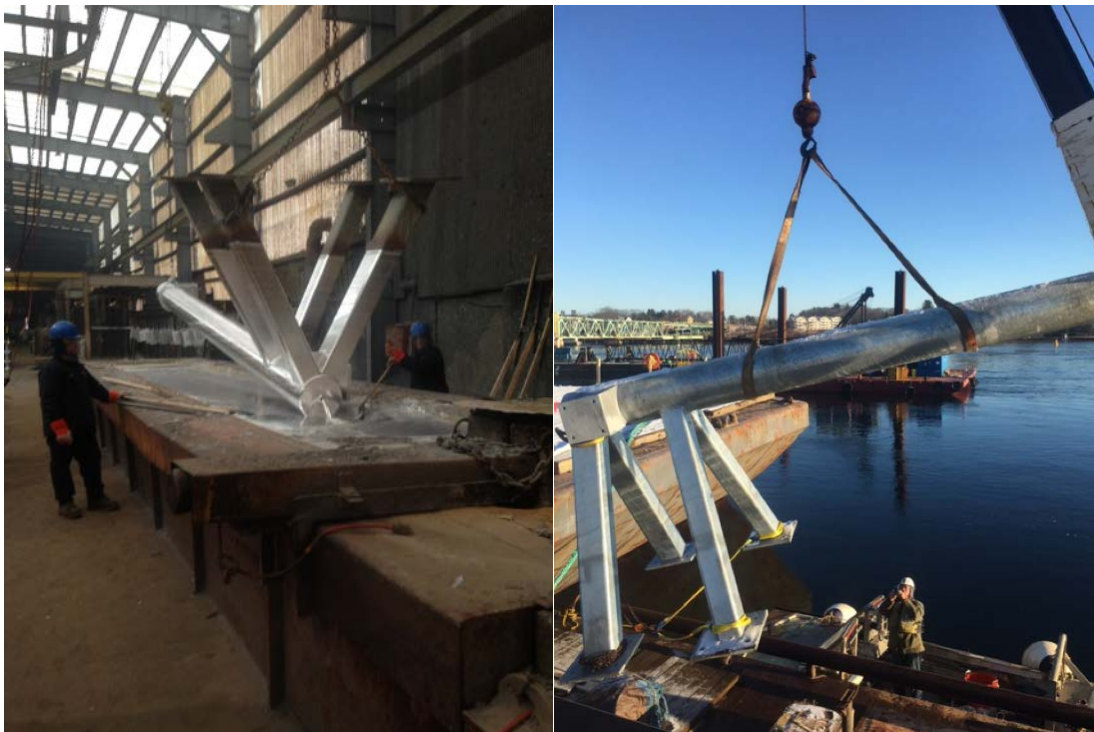
Figure 57. Coating and installation of the VGPs.
