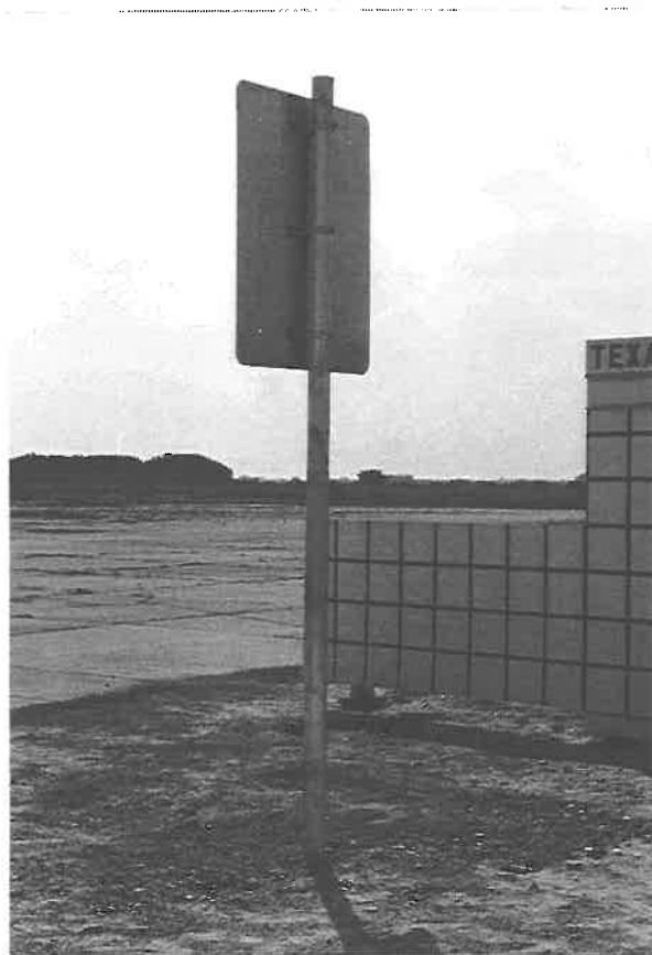
Figure 50 . Single 4 in. aluminum sign support installation anchored in strong soil before test 405231-7.
