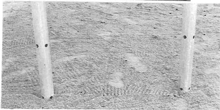
Figure 162 . Dual 4-in with 1-in holes aluminum sign support anchored in weak soil before test 405231-25.
