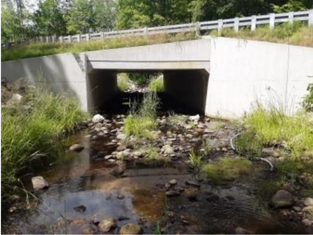
Figure 5: Outlet of Gilford Culvert, performing adequately at low flow conditions
