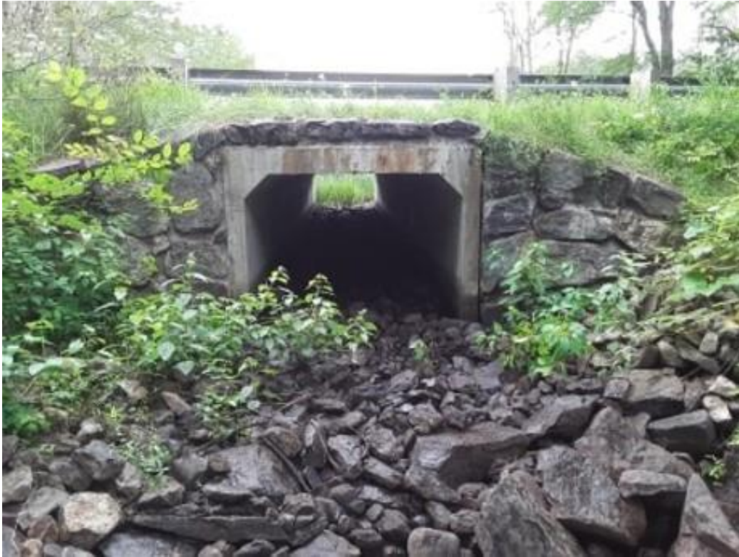
Figure 7: Outlet of Londonderry, Wiley Hill Road Culvert, in hyporheic conditions
