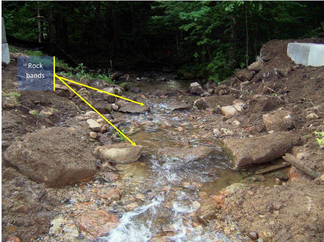
Figure 22: Streambed with rock bands prior to setting bridge deck
