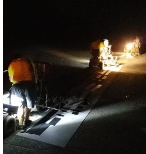
Figure 12: Paint and Bead Application Equipment Calibration
