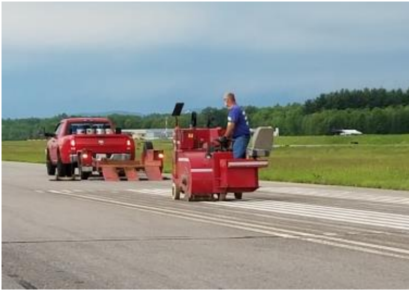
Figure 10: Runway Paint Removal
