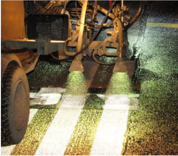
Figure 11: Paint and Bead Installation
