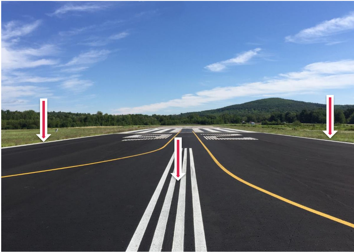
Figure 8: Relationship of Runway Centerline to Edge Stripes
