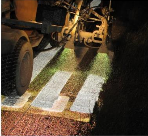
Picture 1 – glass beads spreading too wide.
