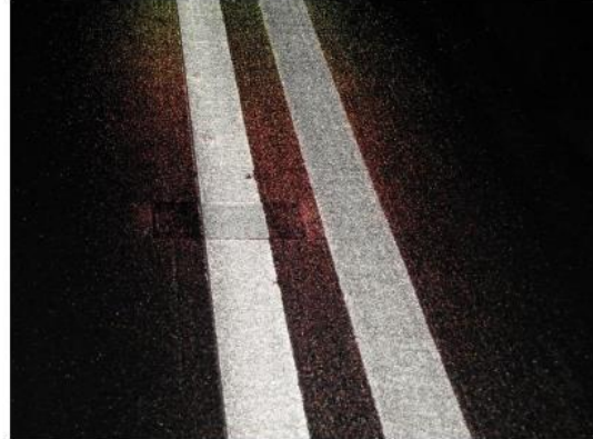
Picture 4 – glass beads applied over line.
