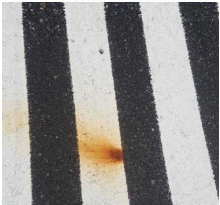
Figure 2: Bottom-up Rust Spot Stain Counting
