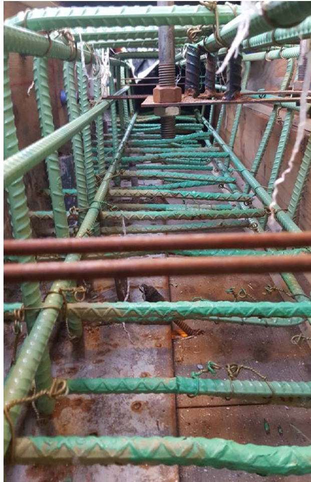
Figure 5: Curb formwork and reinforcement on a curb replacement project.
