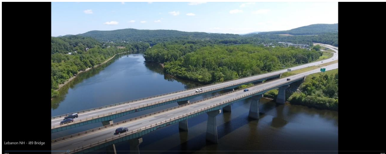
Figure 20. Screen capture of the video created for the bridge inspection case study.
