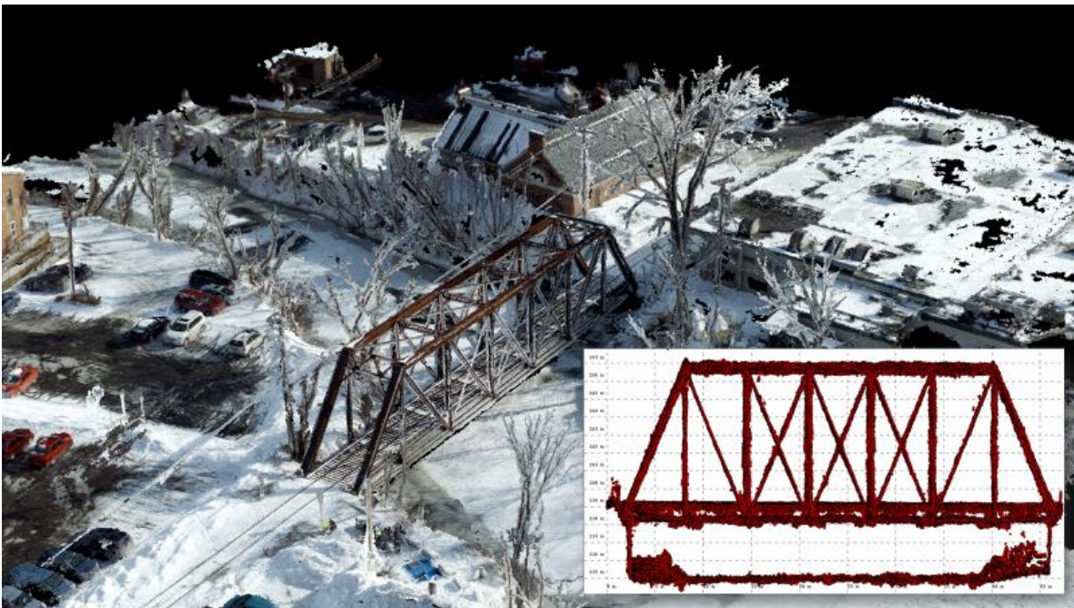
Figure 11. Detailed 3D model of a railroad bridge generated by the senseFly Albris during an autonomous flight operation.
