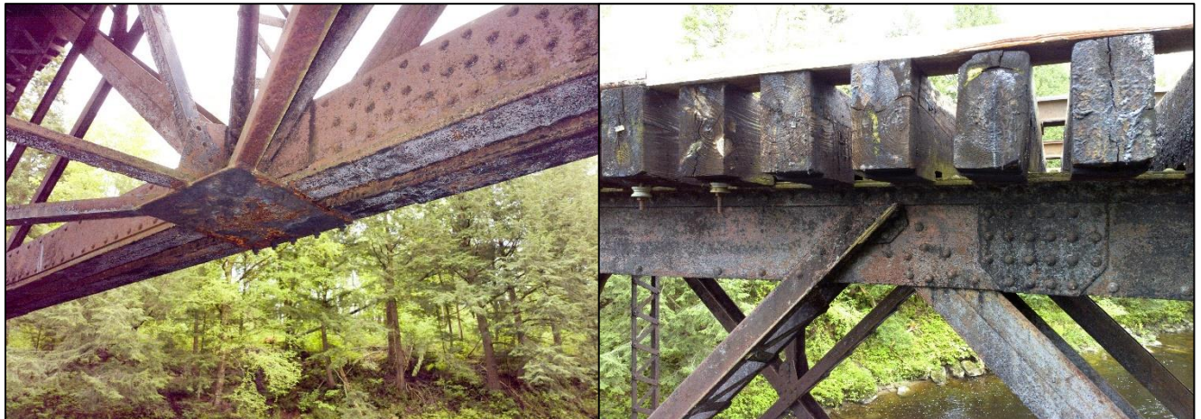
Figure 38. High-resolution inspection photos captured during this case study. The senseFly Albris UAS is able to collect true color photos and videos in addition to thermal images.
