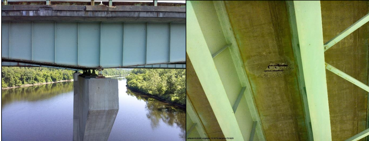
Figure 22. High resolution inspection photos acquired during the bridge inspection case study
