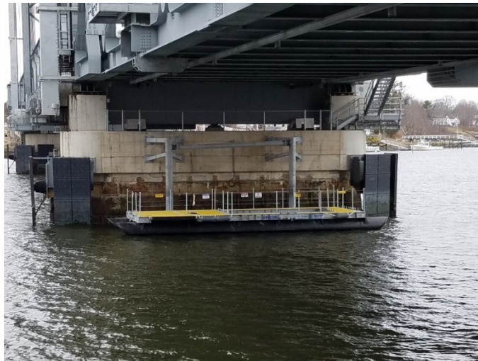
Figure 41. Attachment of the tidal turbine to the Memorial Bridge, NH.
