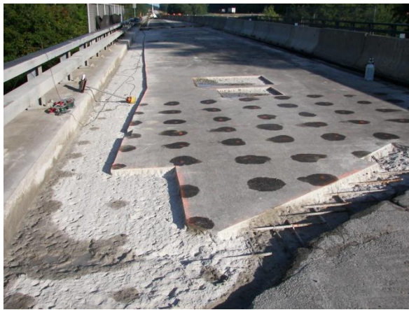
South curb concrete removed
