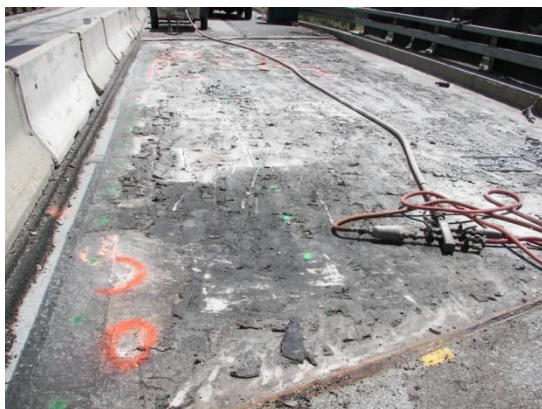
Figure 1. membrane defects
