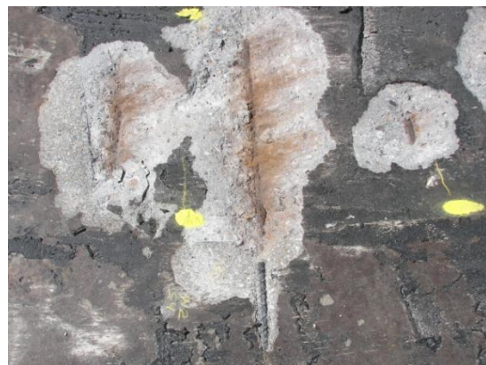
Figure 2. Anodic and cathodic rebar
