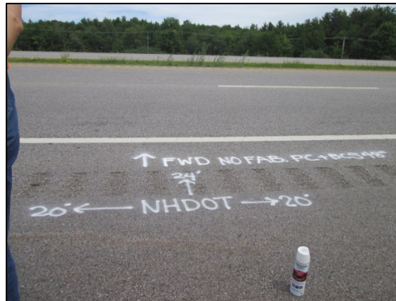
Figure 4. Photographs of the test section in the eastbound travel lane at mile marker 123.3.
