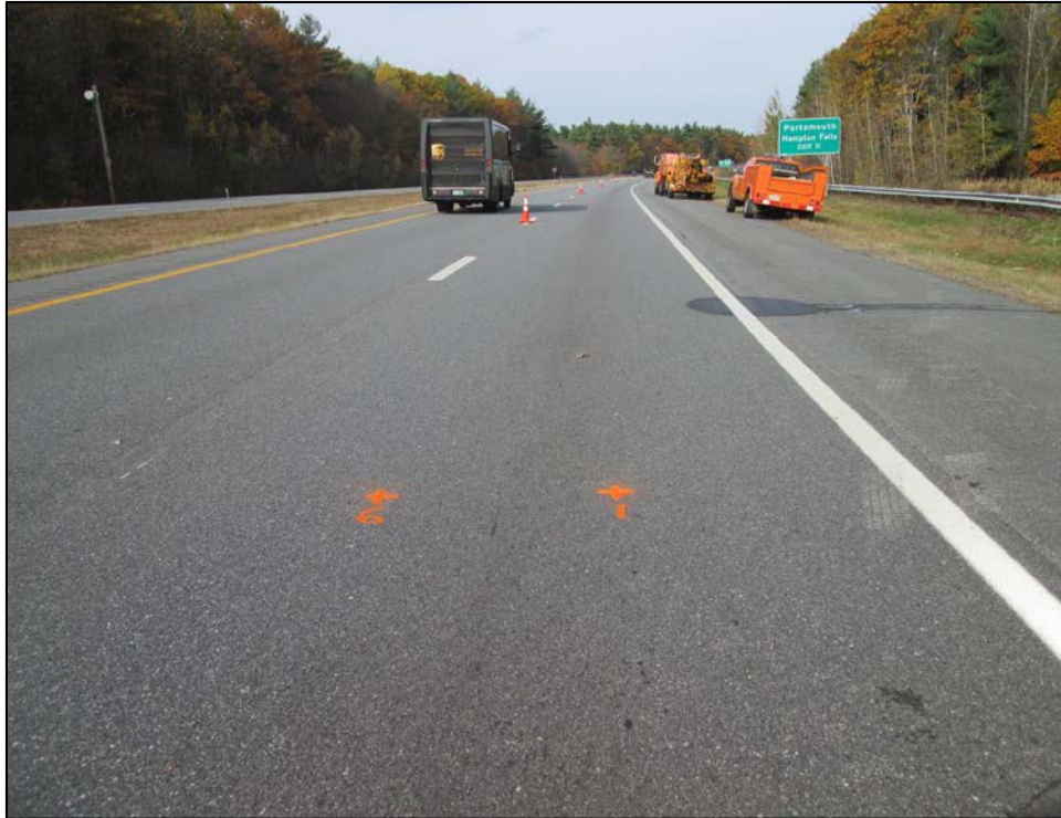
Figure 12. Test section WB MM 128.0 FWD test point locations. The photograph shows the two test points located nearest the core hole: one in the wheel path and six midlane. In this view, the remaining test points continued in the direction of traffic and were spaced approximately 100 ft apart.
