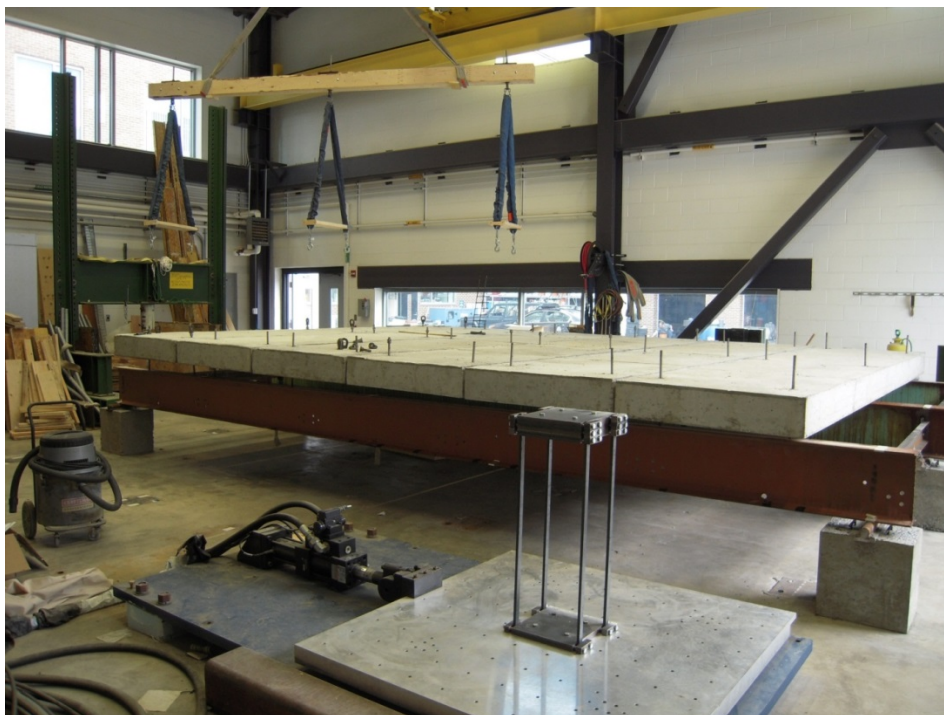
Figure 8 - Full-scale constructability test at UNH.
