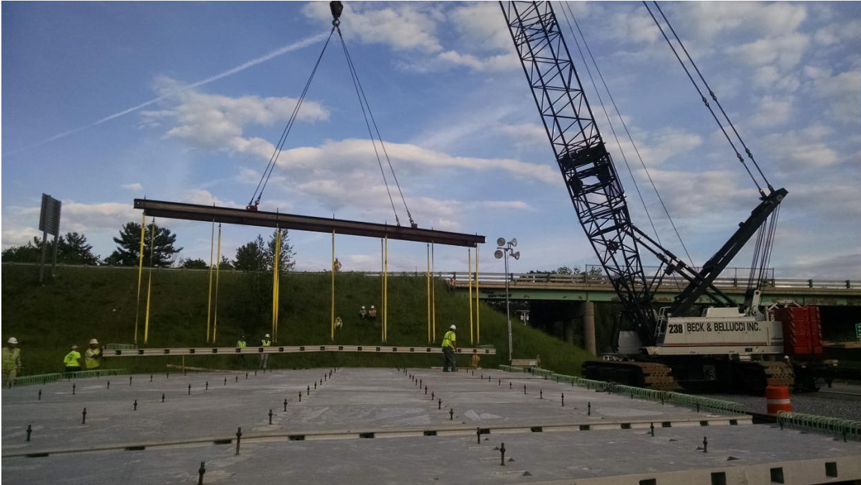
Figure 16 - Loading out Panel 1.
