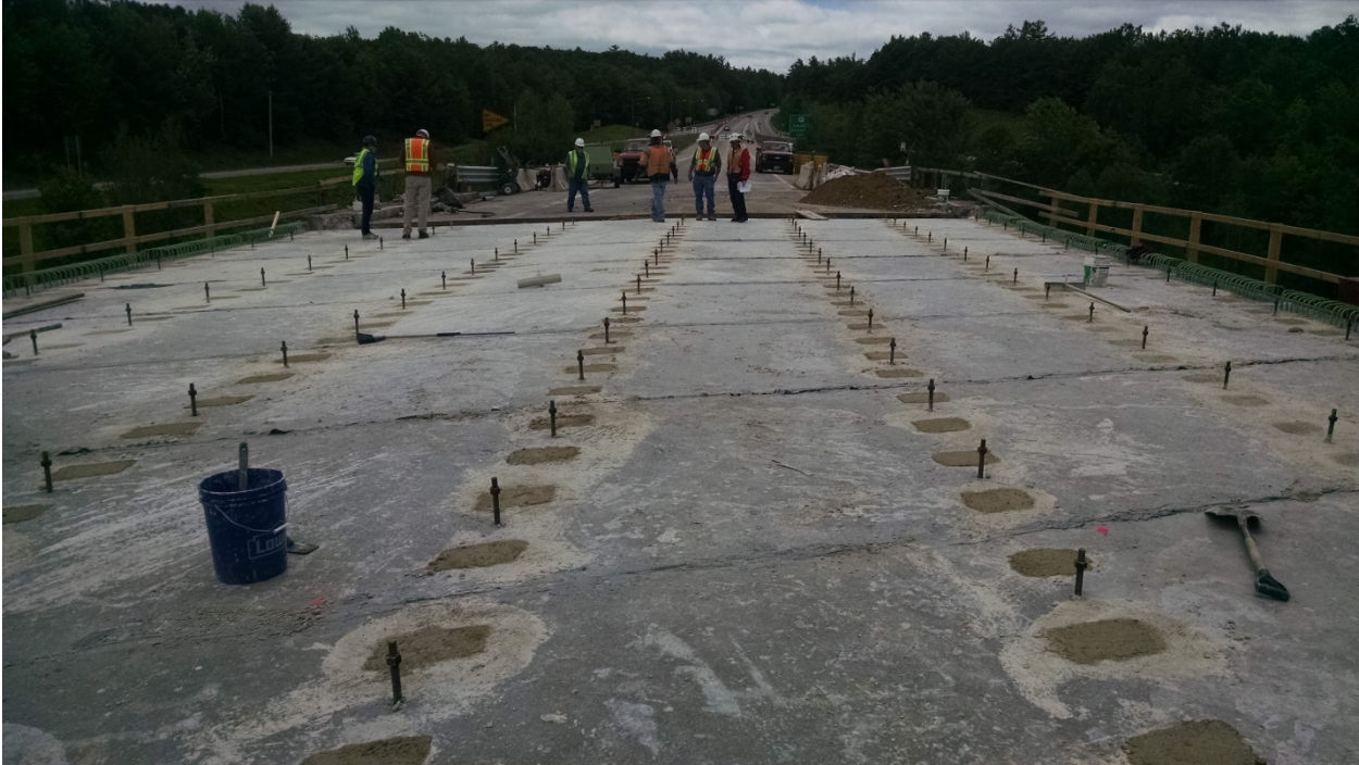
Figure 28 - Deck following shear connector and haunch grouting.
