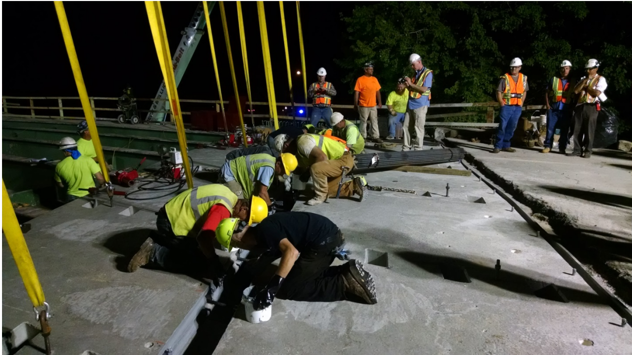
Figure 20 - Applying mixed polymer along Joint 1.
