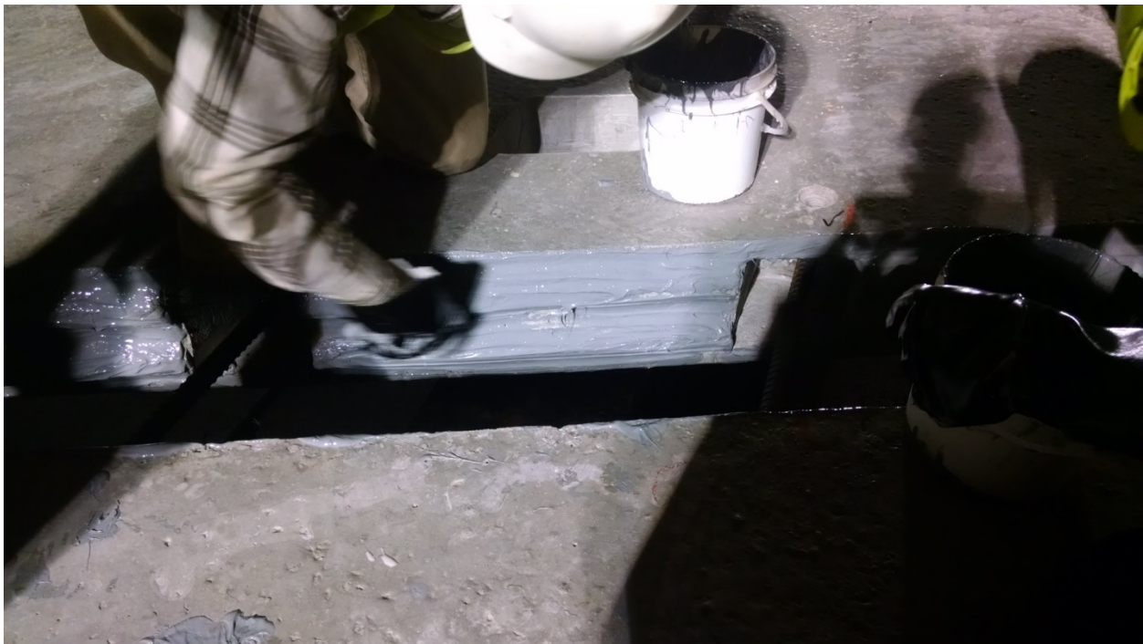
Figure 21 - Typical polymer application by hand.
