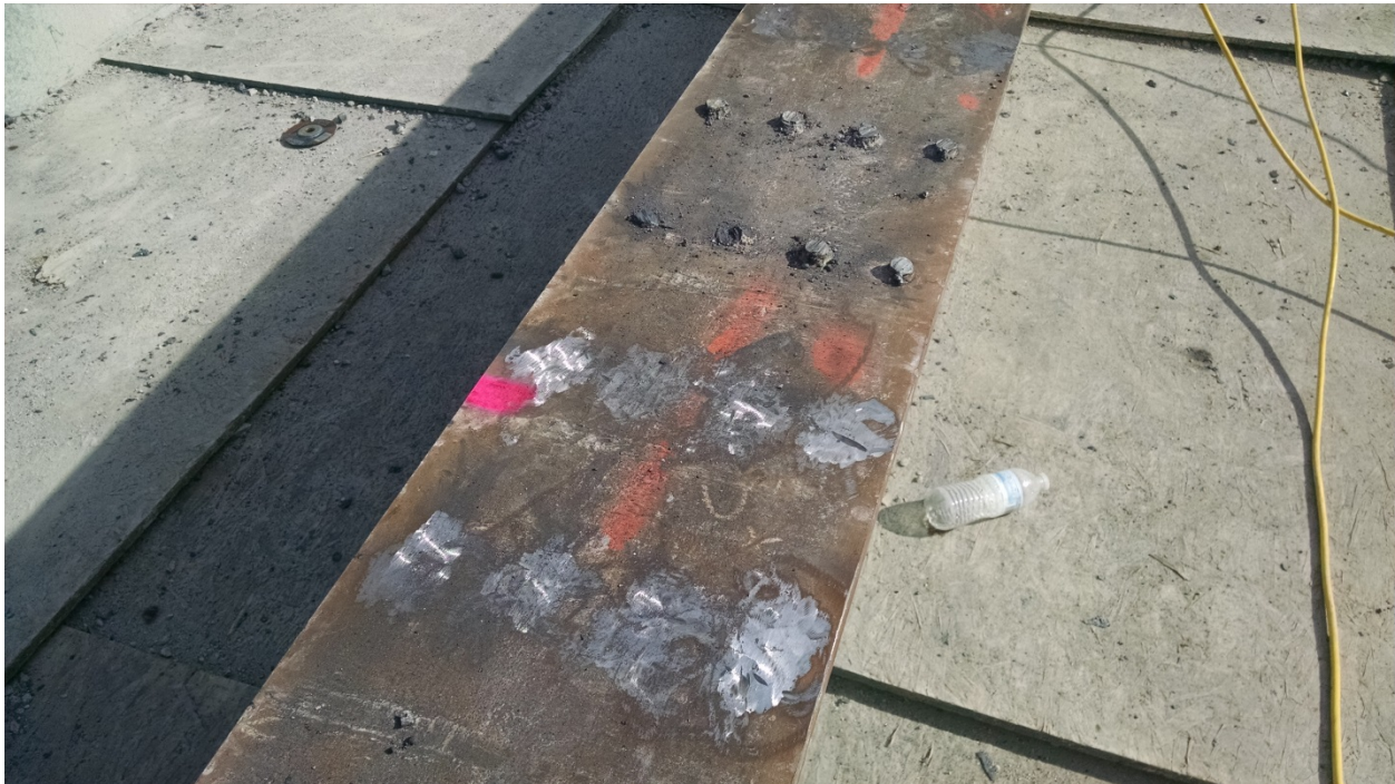
Figure 14 - Leveling screw location preparation.
