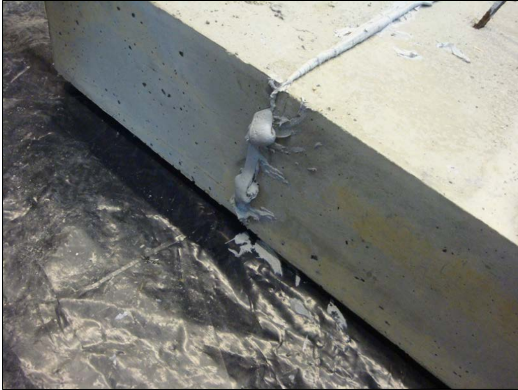
Figure 1 - Polymer forced out of a tested joint following initial joint stressing.
