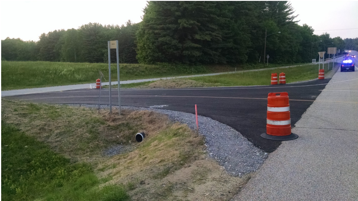
Figure 30 - Crossover between an off-ramp (l) and US 3 (r) with traffic flow to the left.
