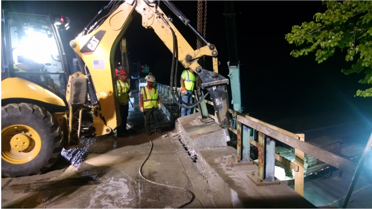
Figure 10 - Segmental coping demolition.
