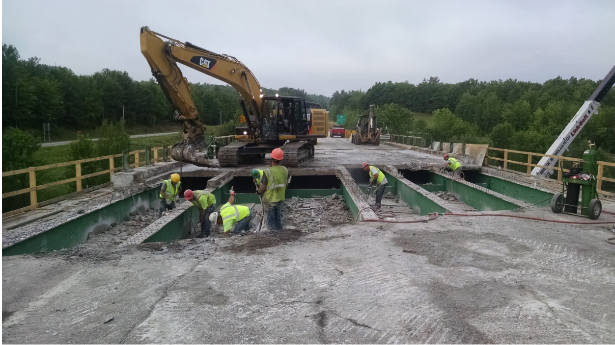
Figure 13 - Deck removal nearing halfway point.
