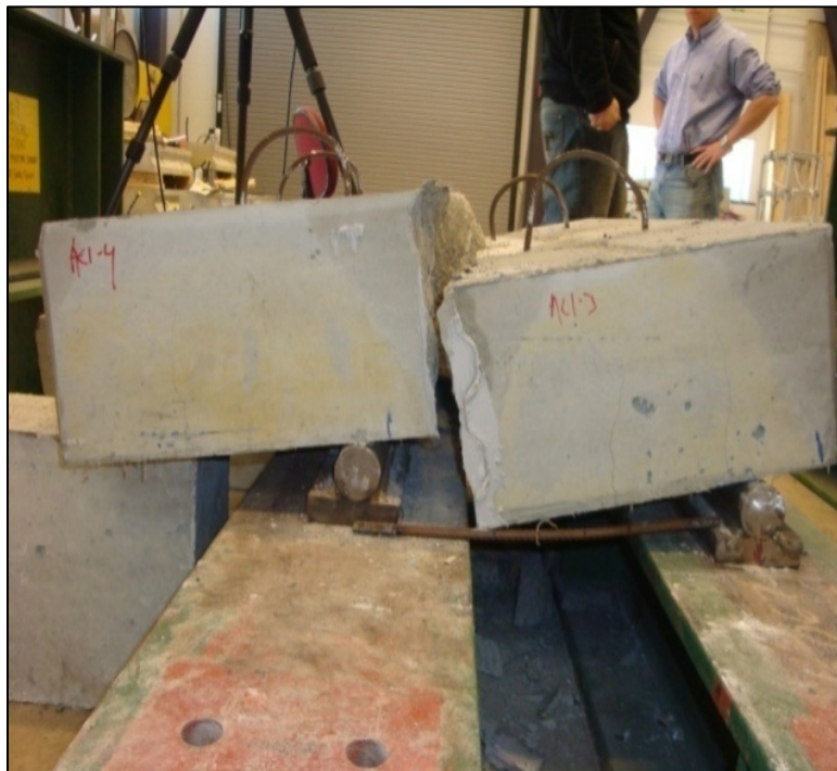
Figure 2 - Tested joint showing failure behind the sealed joint.
