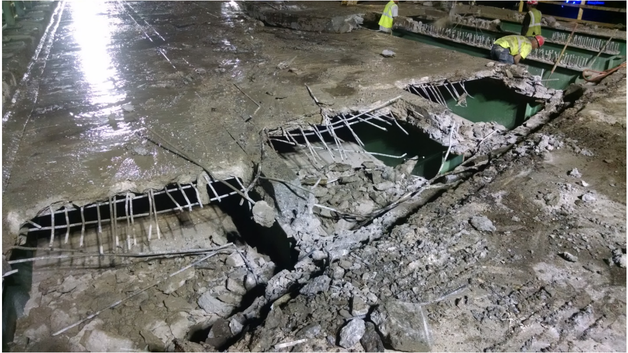
Figure 11 - North deck end demolition.
