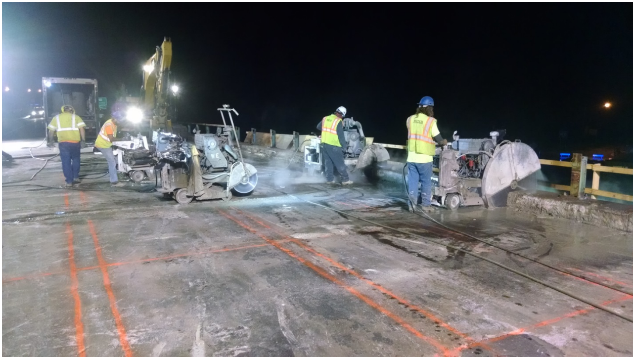
Figure 9 - Sawcutting in progress showing slab layout.
