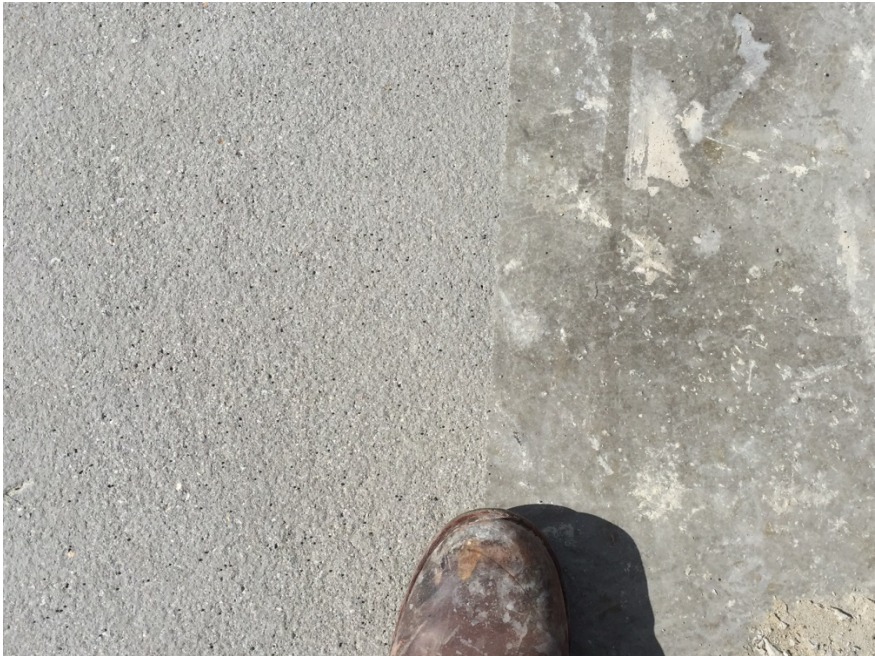
Figure 29 – Sandblasted (l) versus non-sandblasted (r) deck surface.
