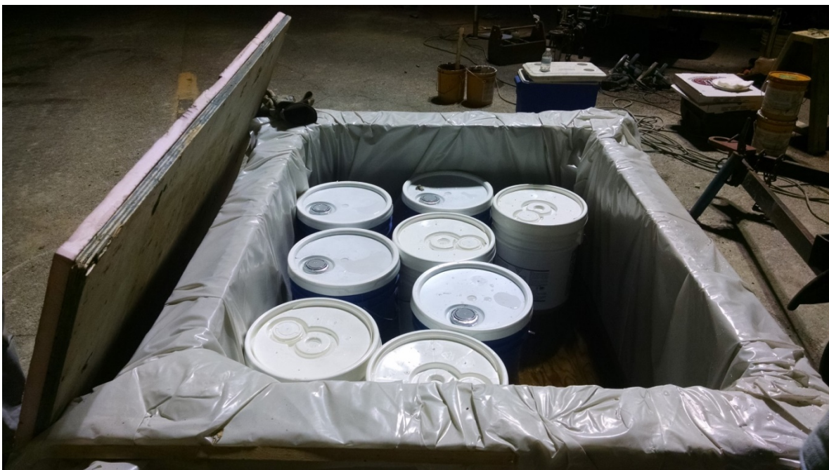
Figure 19 - Polymer component cold storage on site.
