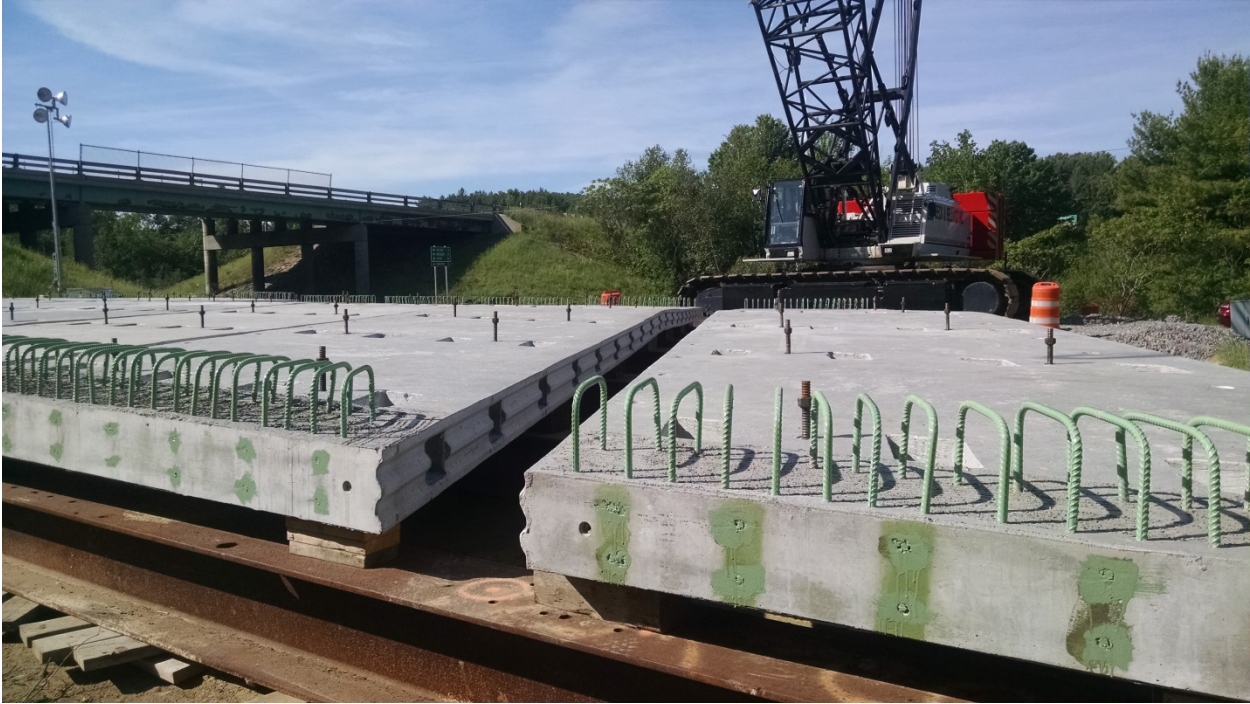
Figure 15 - Panels staged on blocking prior to erection.
