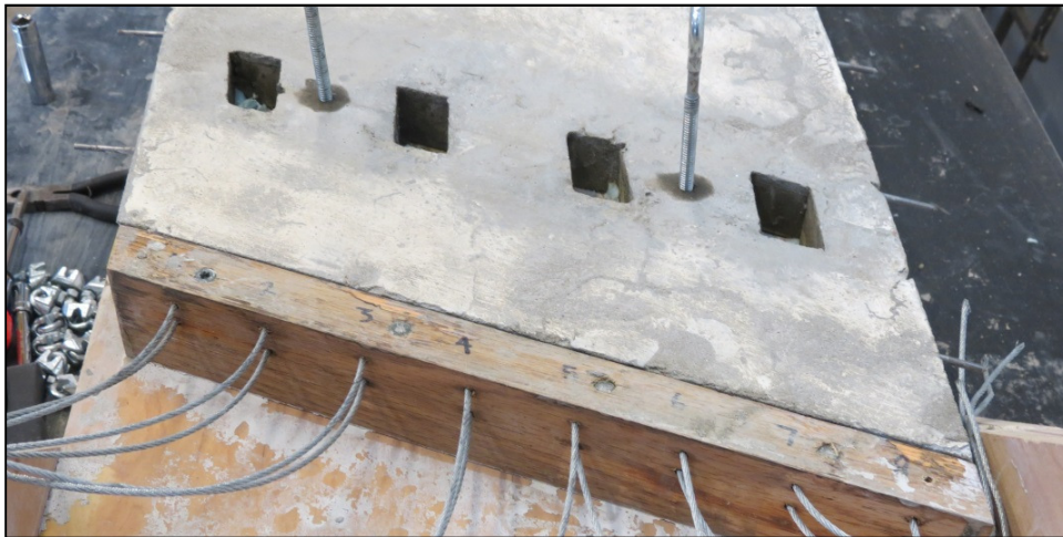
Figure 16: Releasing the Prestressing Cables
