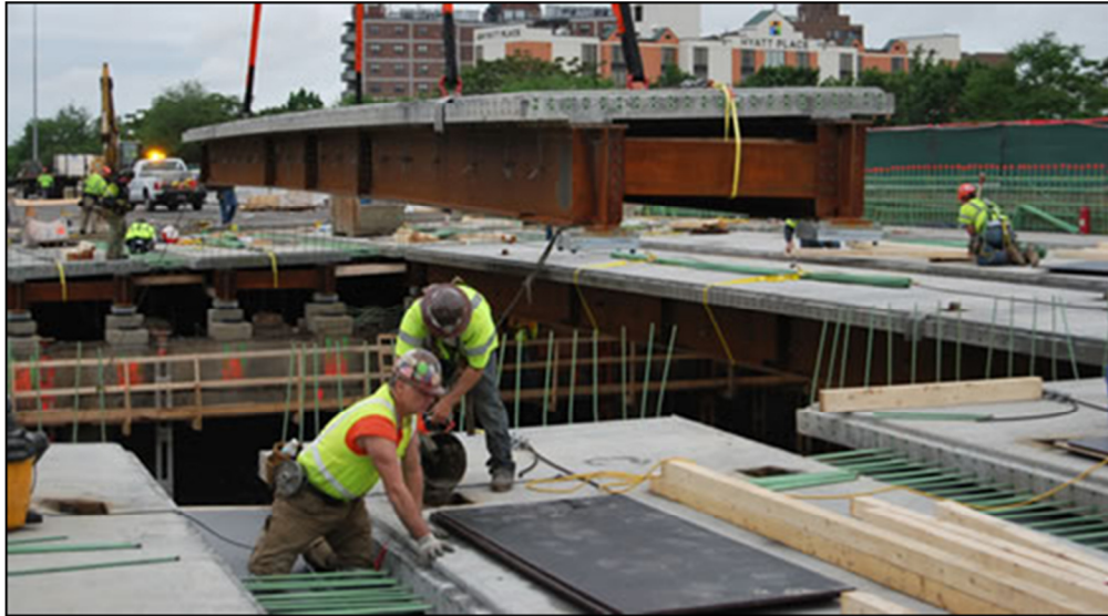
Figure 1: Zipper Pours - Massachusetts Fast 14
