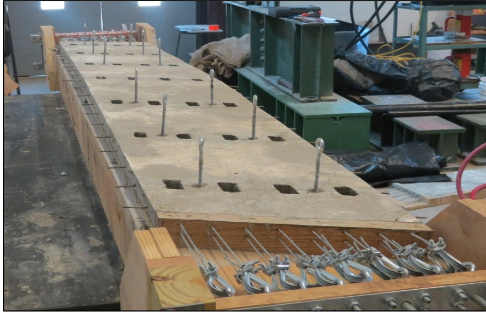
Figure 15: Full Slab after Stripping
