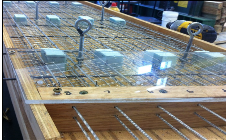
Figure 13: End of Slab Form
