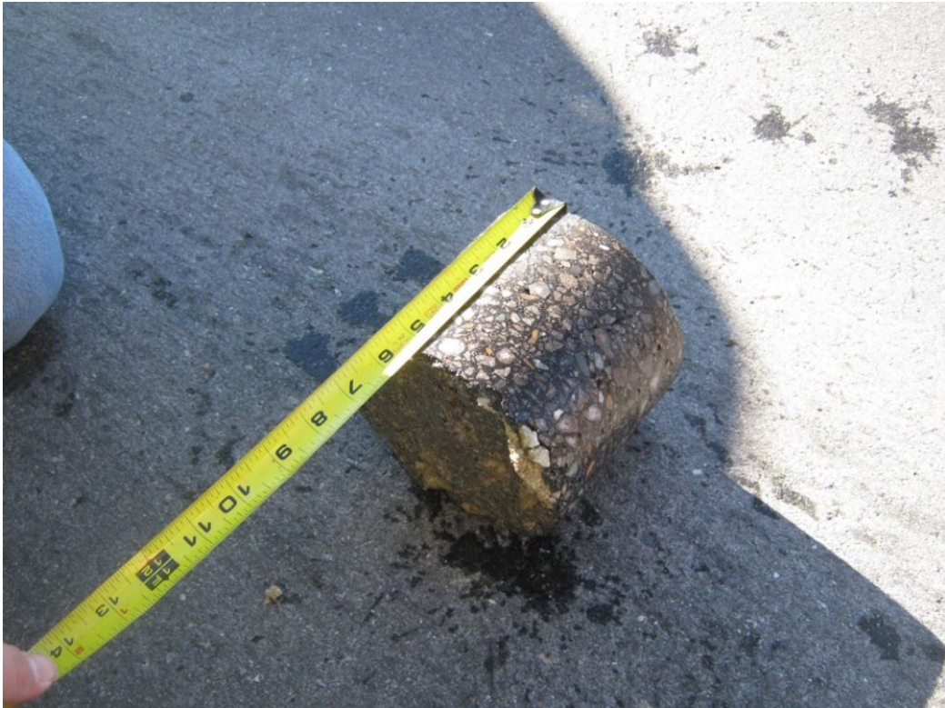
Figure 4. Cored asphalt concrete at location FT5.
