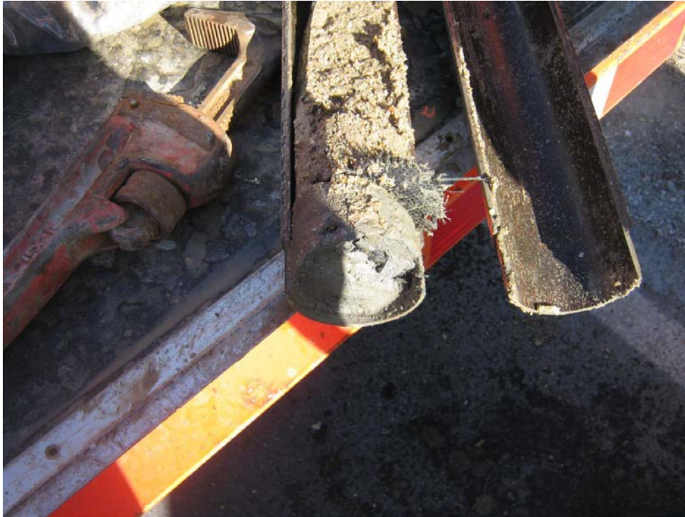
Figure 5. A core of base materials through the geotextile and down to the subgrade at location FT1. The light brown sand subbase material is above the geotextile and natural gray sandy silt subgrade material.
