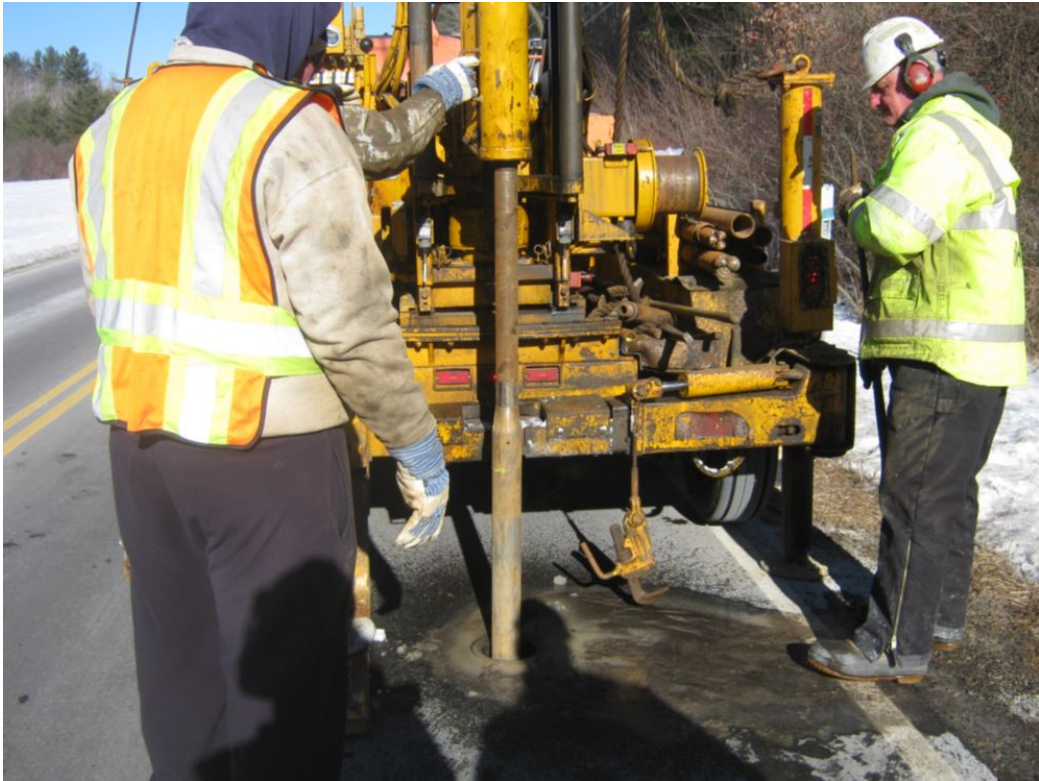
Figure 3. Coring operation and sample collection.
