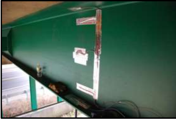
Figure C-17: Photo of Gauge Installation – Aluminum Tape Environmentally Protecting
