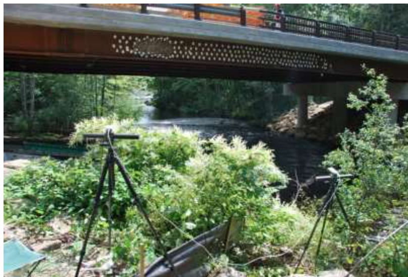
Figure F-11: Cameras not setup level with girders. Note: this photo is of previous research performed at UNH.
