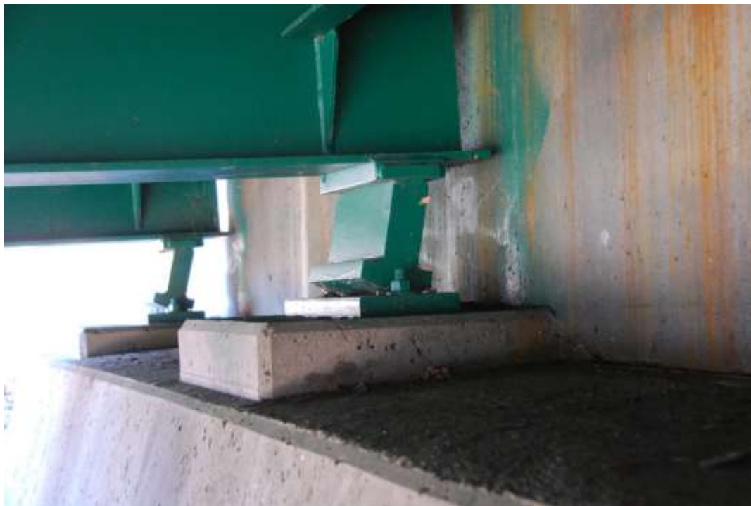
Figure 60: Fully tipped rocker bearings at North Abutment.
