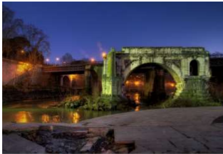
Figure 1: Surviving center span of Pons Aemilius Rome, Italy (credit: Flickr.com).
