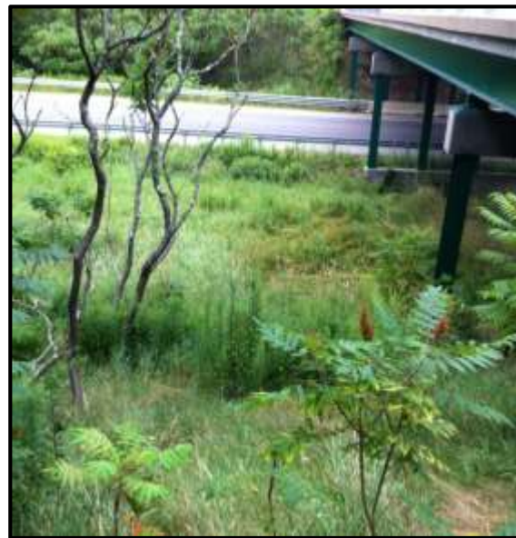
Figure C-2: Photo of Sloped Terrain and Vegetation Growing Around Eastern Abutment at BRB
