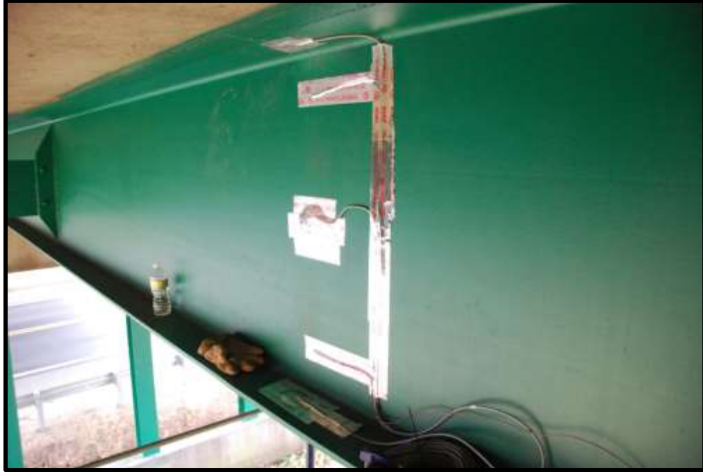
Figure G-13: Photo of Taped Sensor on South Face of Beam D, Showing Thermocouples
