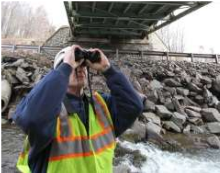
Figure 66: PennDOT inspector assesses an abutment using binoculars during a Routine Inspection (Scranton Times Tribune).
