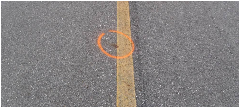
Photo 1—Proposed core location 1. Locations west of taxiway intersection.
