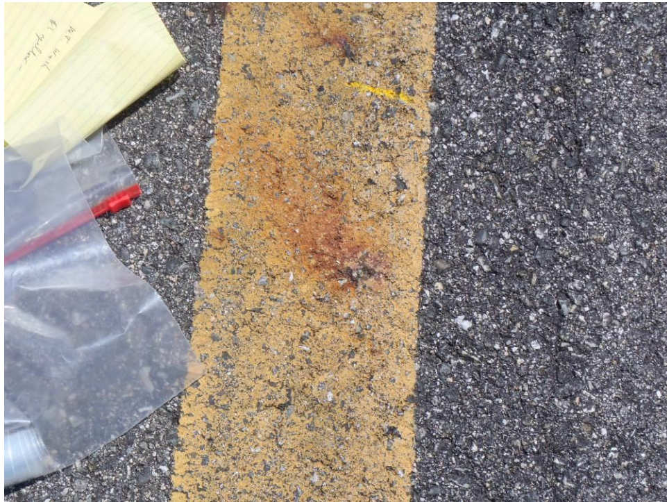
Photo 2 – Close up of paint sample location 1 before sampling.
