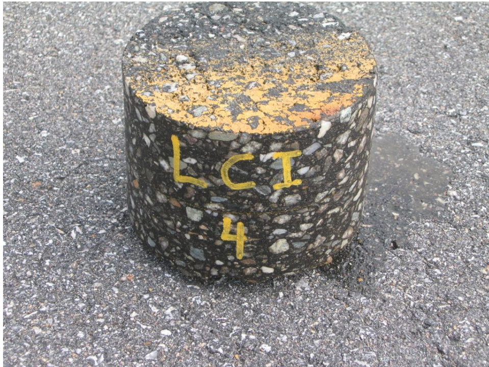
Photo 14 LCI Core 4 - taxiway C centerline across from terminal apron
