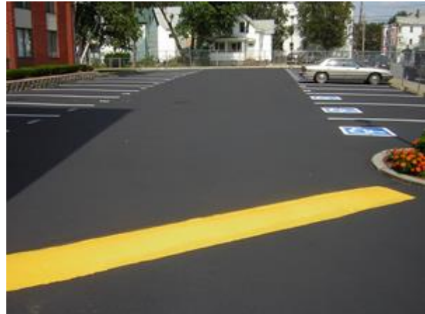
Figure 18 - Sealed and painted pavement
