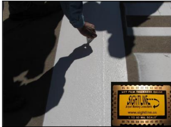
Figure 17 – Paint thickness measurements and Mil Thickness measuring tool -lower right (Speidel 2014)
