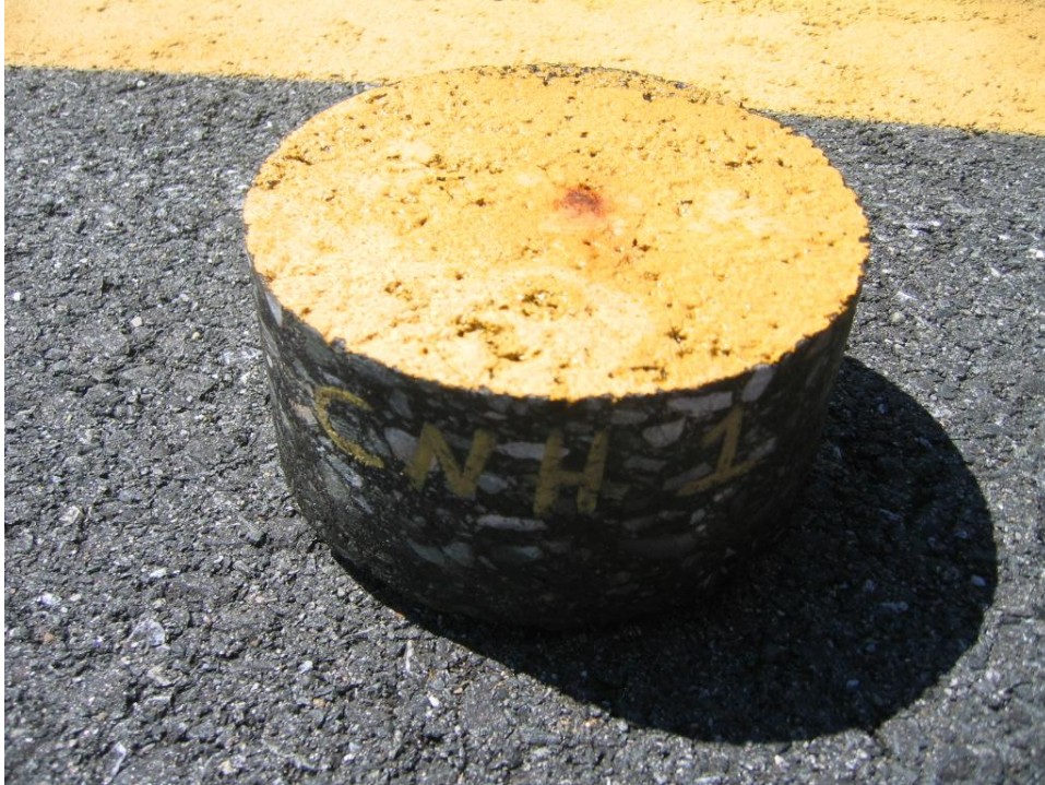
Photo 10 – Claremont Municipal Airport (CNH) Core 1 – east end of taxiway C (west)
