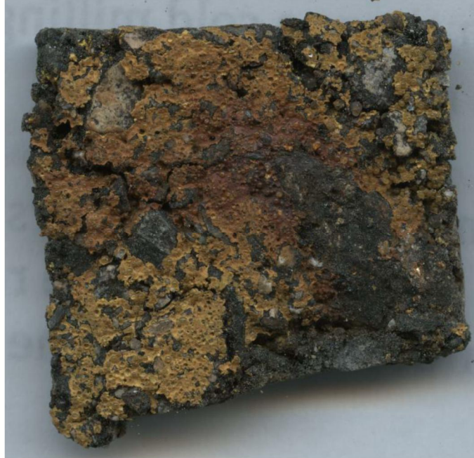
Figure 22 Whitefield paint chip showing source of iron staining
