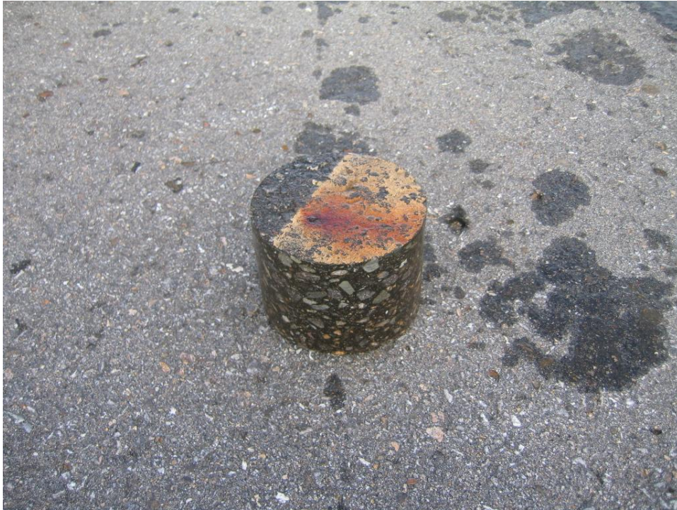
Photo 11 Laconia Airport (LCI) Core 1 - blast pad left side runway 8 end
