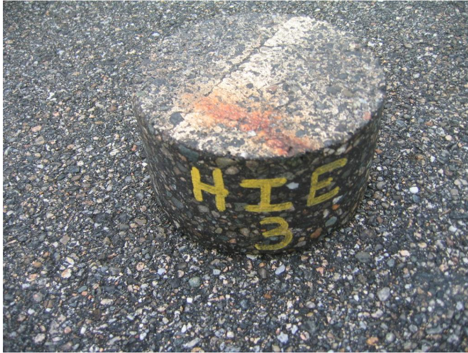
Photo 16 - HIE Core 3 from tough down marking runway 10 end left side.
