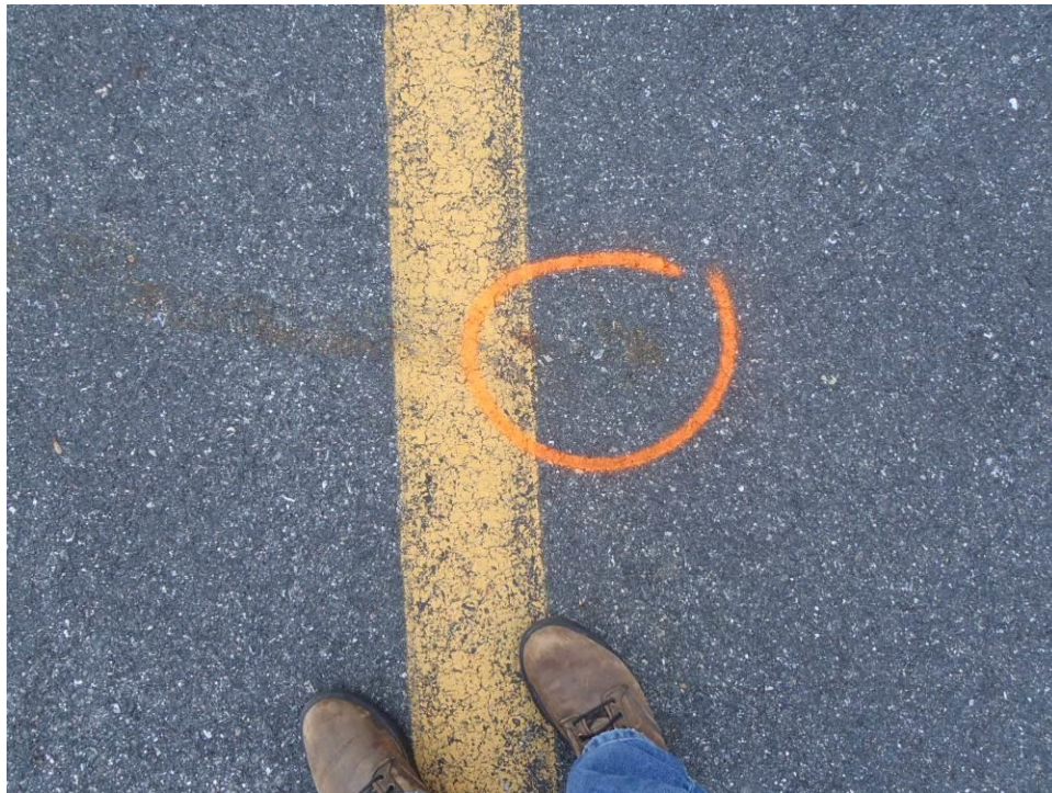
Photo 6 - Close up of proposed core location 2.
