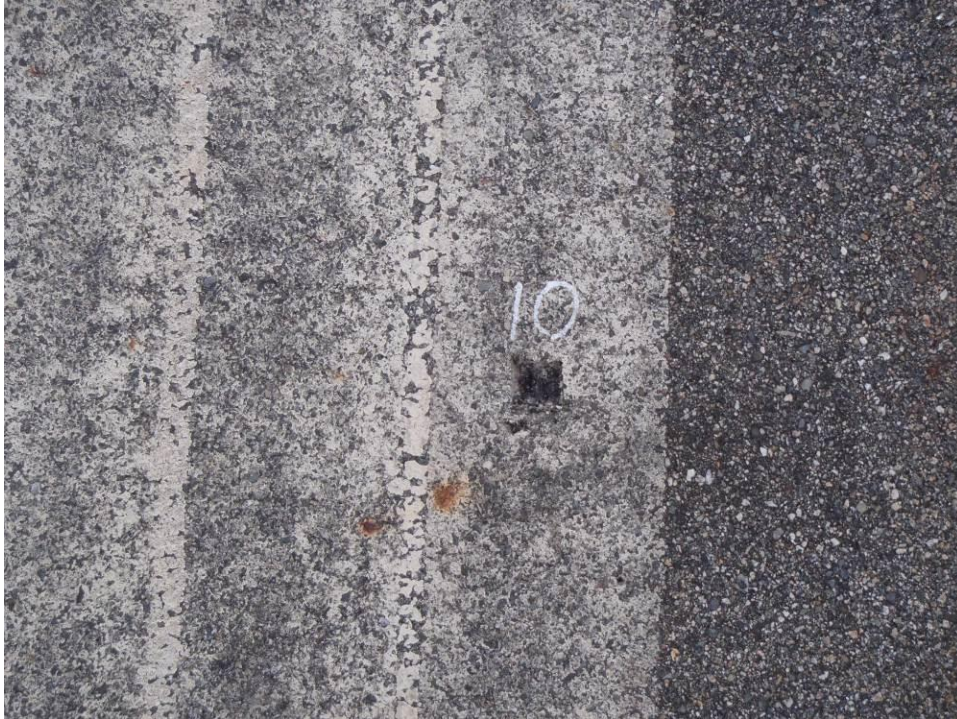
Photo 13 – Close up of paint sample 10 after sample taken.
