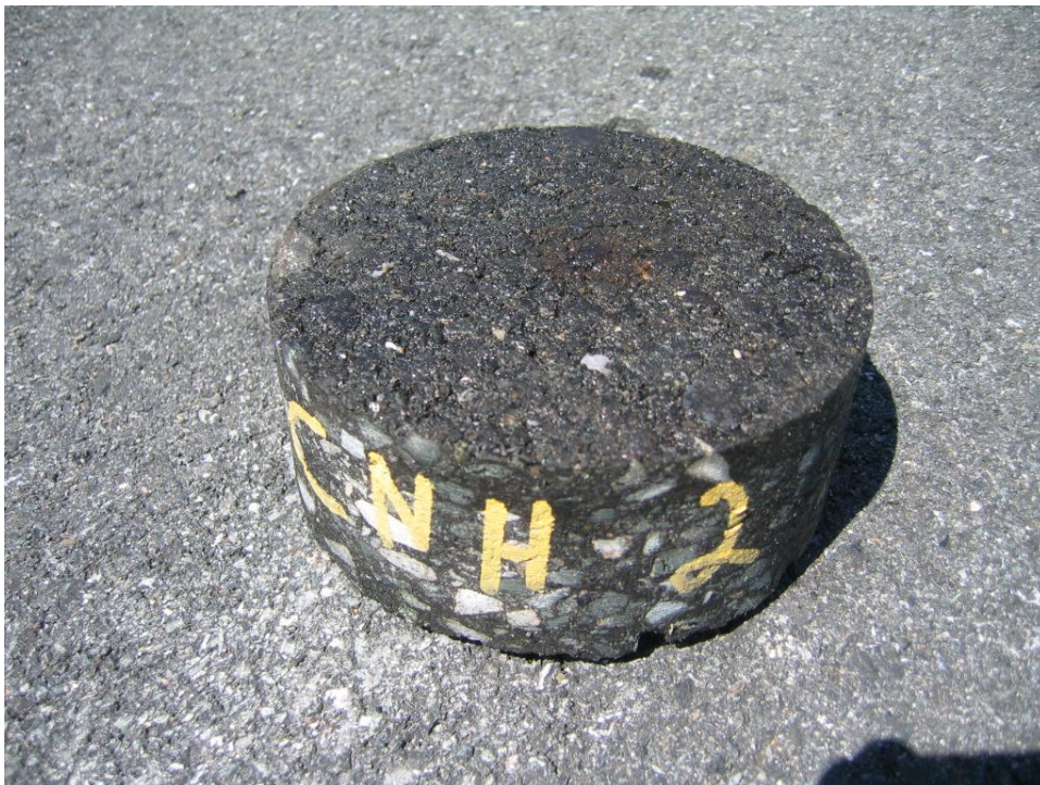
Photo 11 – CNH Core 2 – east of taxiway C (west)
