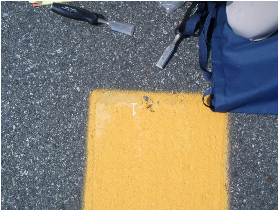
Photo 1 – Close up of paint sample 1. Note only the paint was removed.
