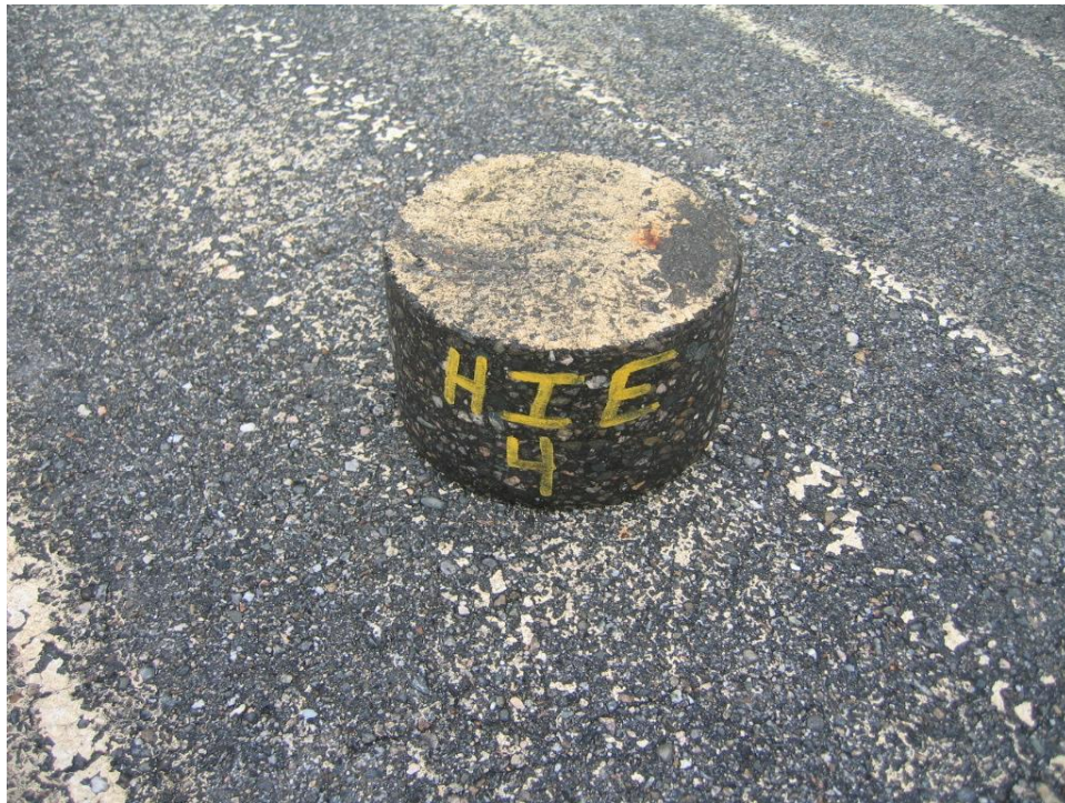
Photo 17 HIE Core 4 from touch down marking runway 10 end right side.
