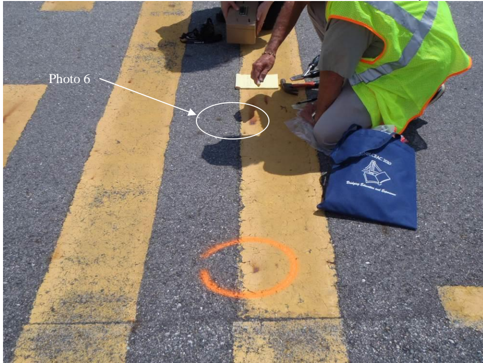
Photo 5 – Proposed core location Western end of taxiway at Hold Line
