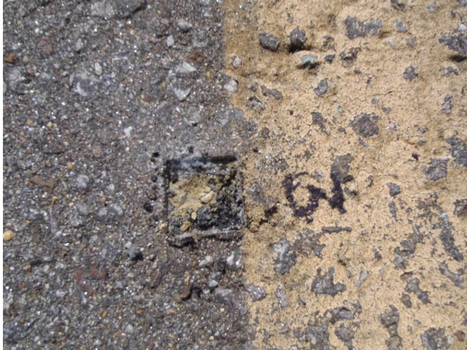
Photo 3 – Close up of sample 3 before removal.
