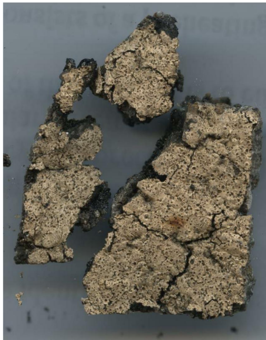
Figure 25 Whitefield paint chip showing small source of staining
