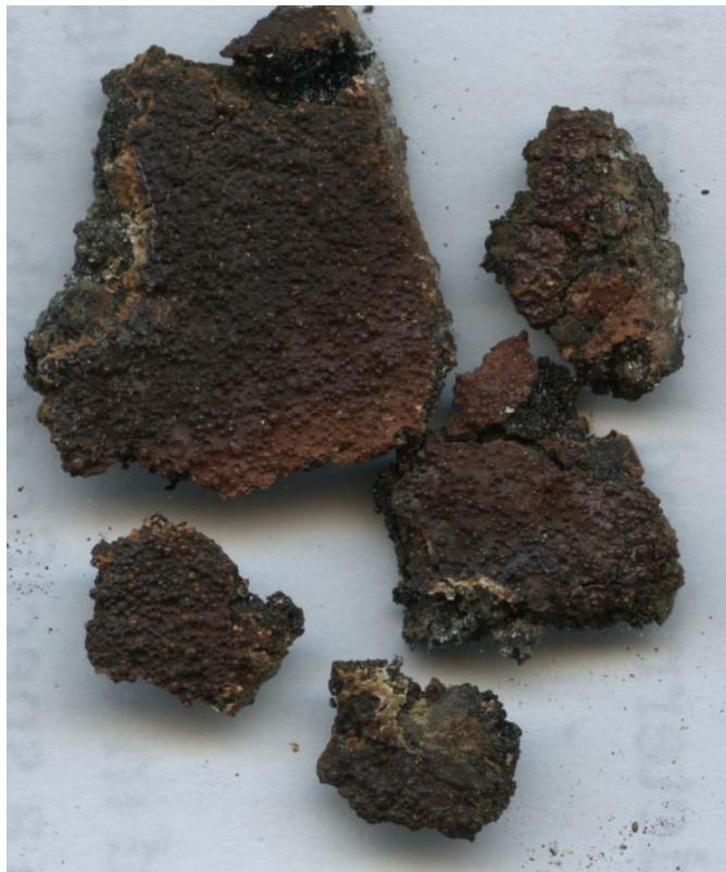
Figure 17 Laconia paint chips showing major iron staining
