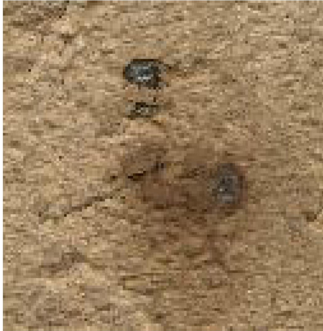
Figure 15 Close up of stained area from Figure 14
