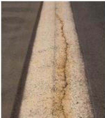
Figure 11 - Stained markings before modified paint (Speidel, 2008)
