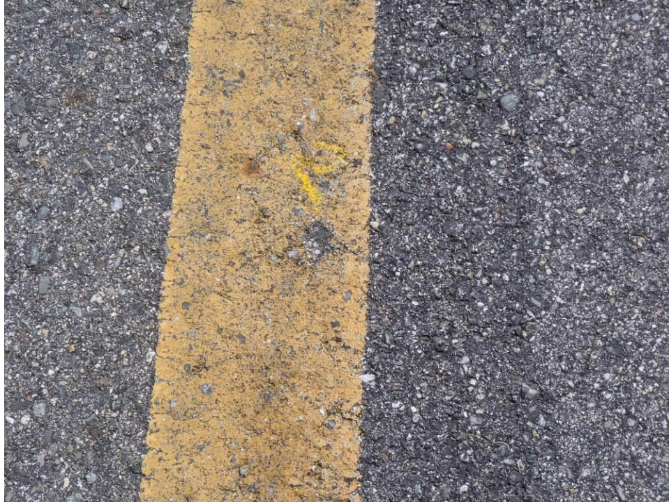
Photo 3 – Close up of paint sample location 2 before sampling.
