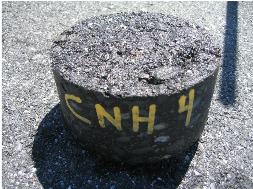
Photo 13 – CNH Core 4 - west end of taxiway C (east)
