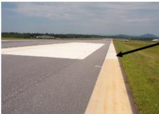
Figure 20 – Grooved Pavement Example (white with black arrow) and not grooved (stained) pavement (Speidel 2008)
