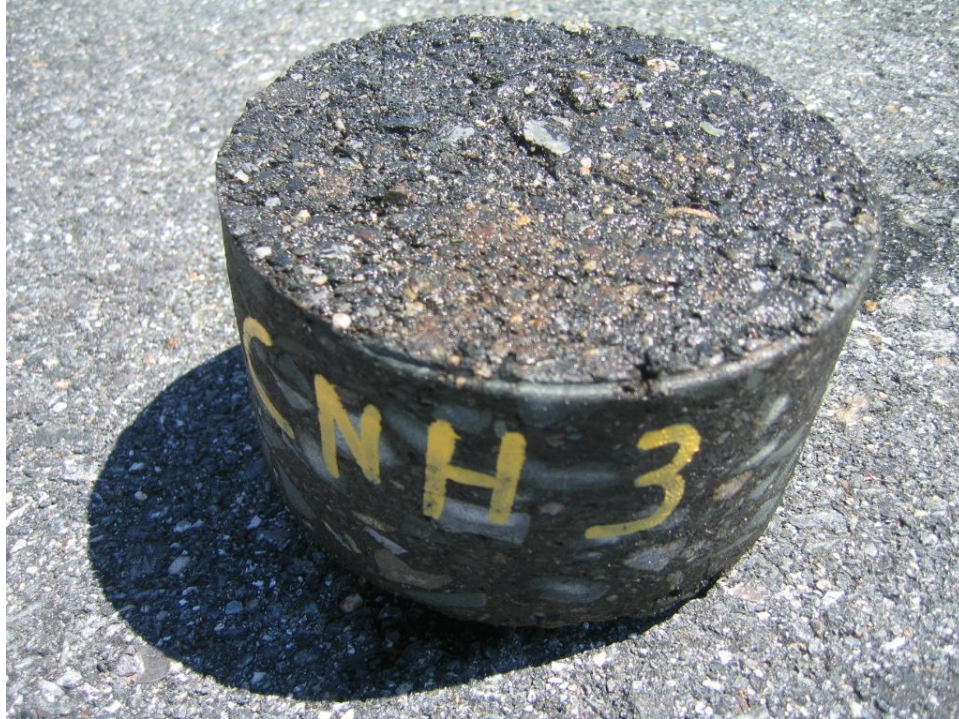
Photo 12 – CNH Core 3 - west end of taxiway C (east)
