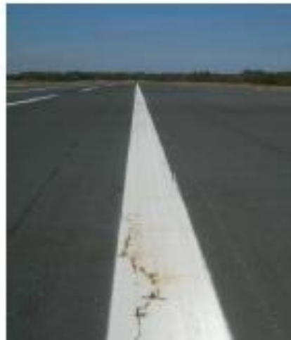
Figure 12 - Modified paint 2 years after (Speidel, 2008)
