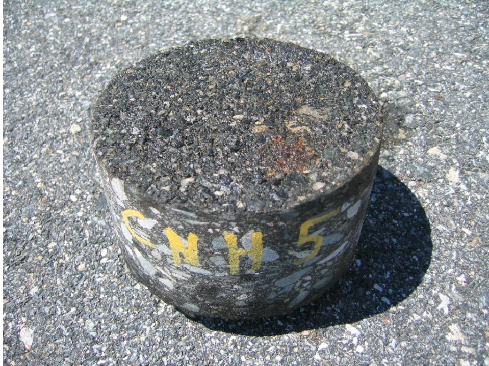
Photo 14 – CNH Core 5 – Hangar Pavement in project AIP 3-33-0002-16-2005 pavement area
