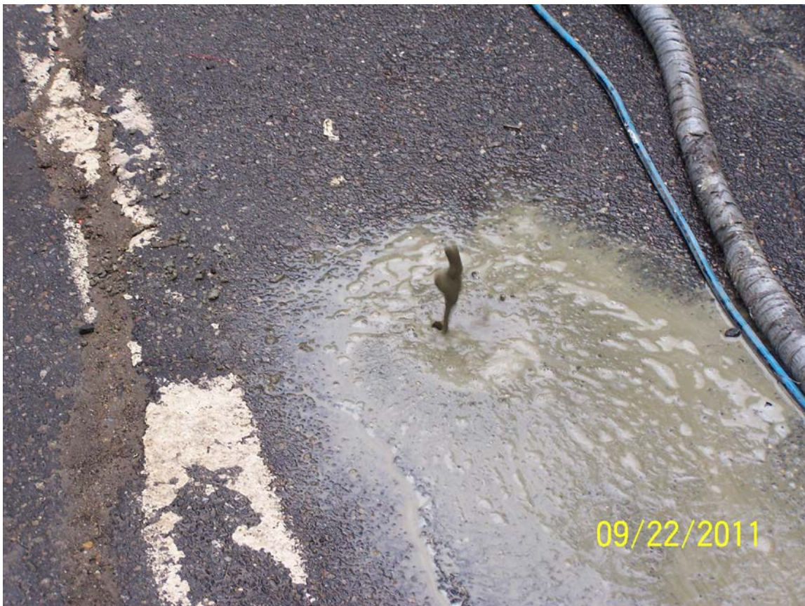
Southbound lane injection forced groundwater to shoot from prepared holes.
