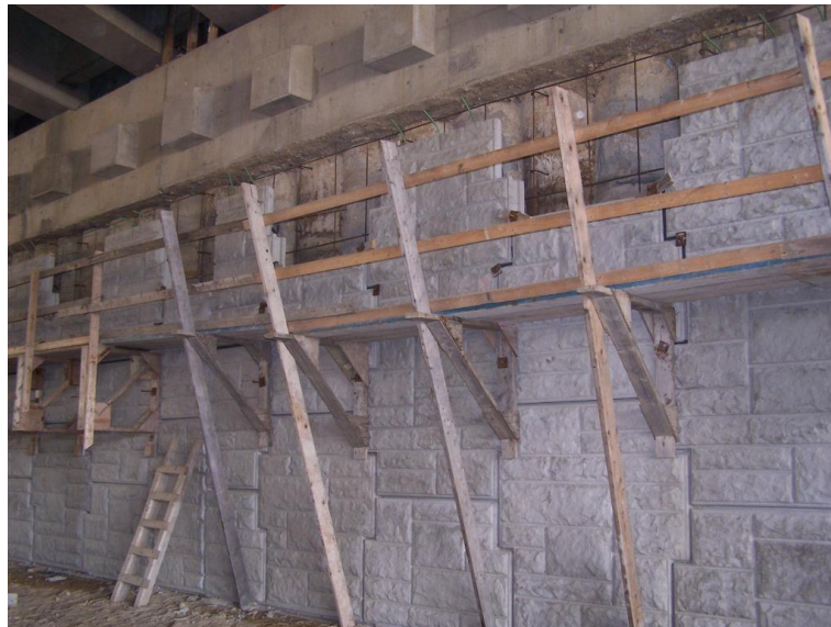
Figure 23: Architectural wall that conceals secant pile wall
