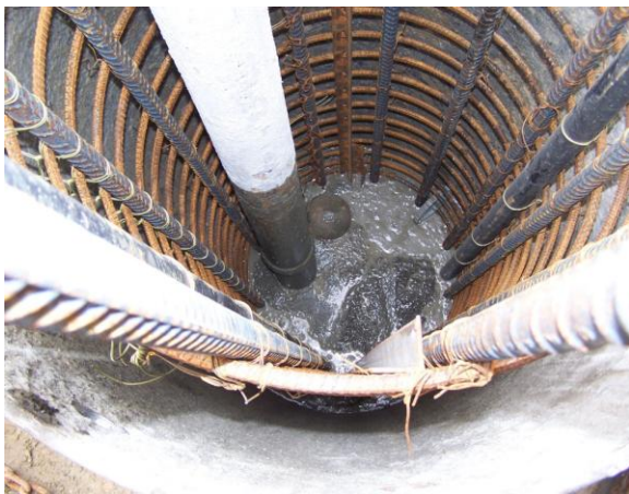
Figure 7: Pumping SCC into Shaft
