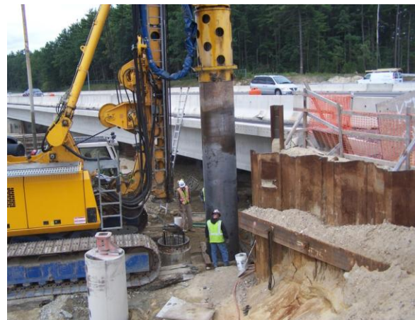
Figure 8: Removing a section of casing
