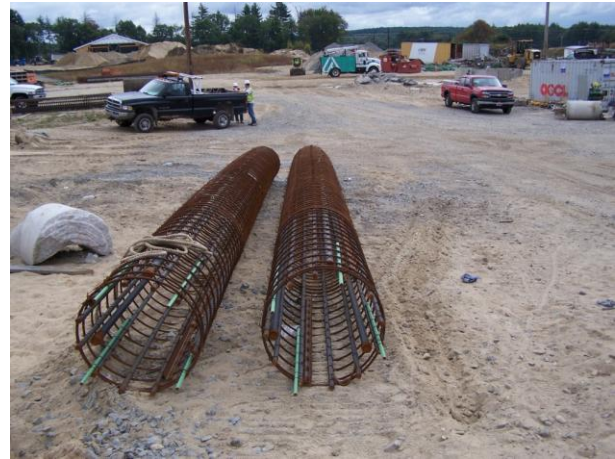
Figure 6: Rebar cages before installation
