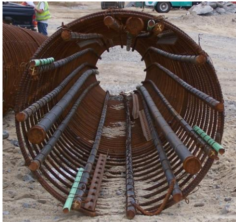
Figure 9: Sonic crosshole logging tubes
