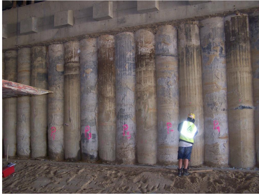
Figure 22: Primary piles are marked in pink paint
