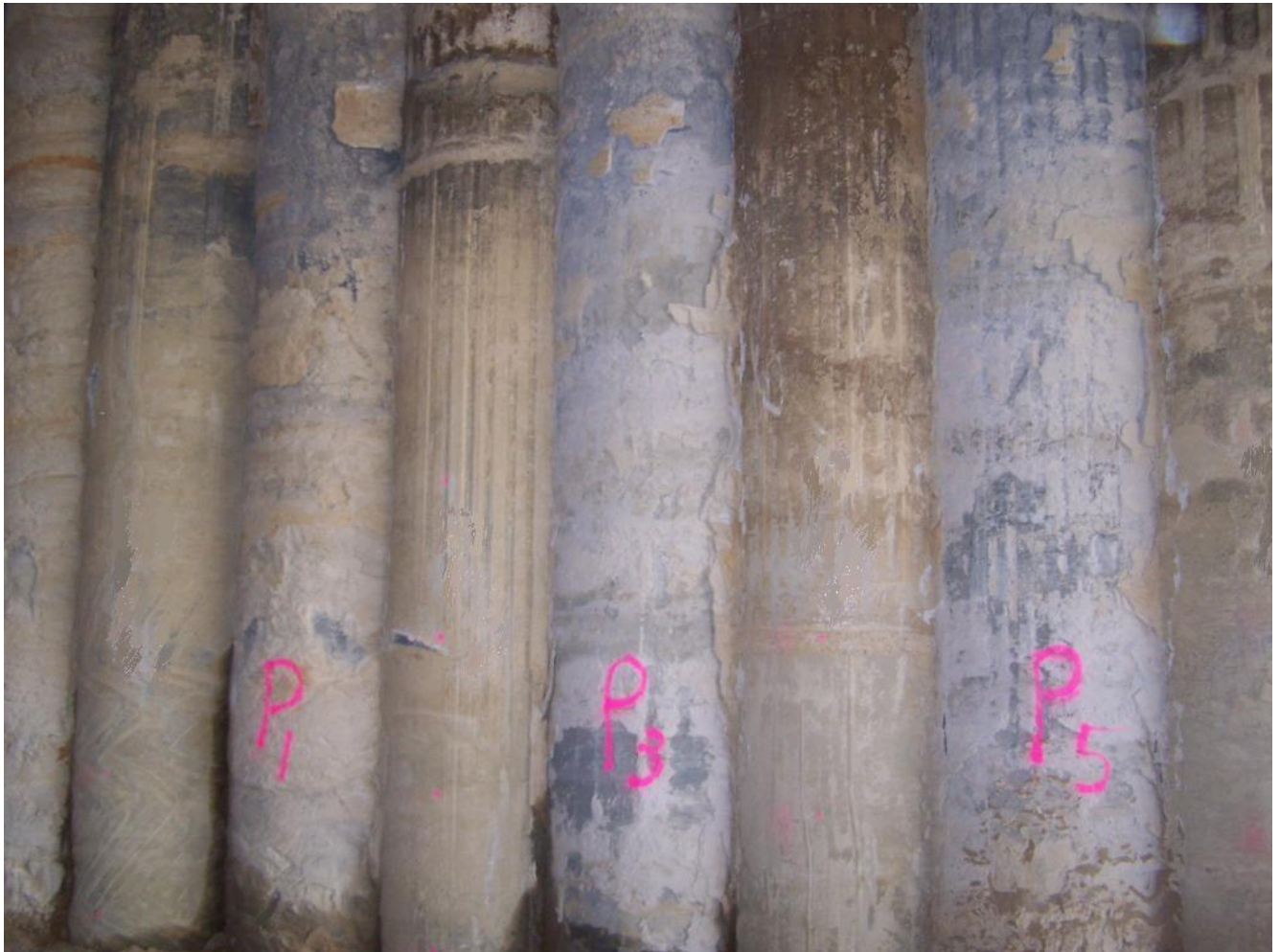
Figure 24: Primary SCC piles N3P1, N3P3, and N3P5
