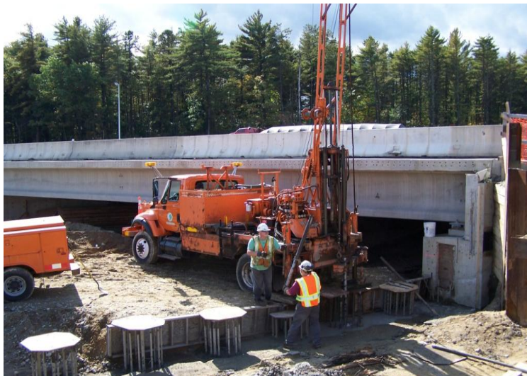
Figure 10: Coring secant piles
