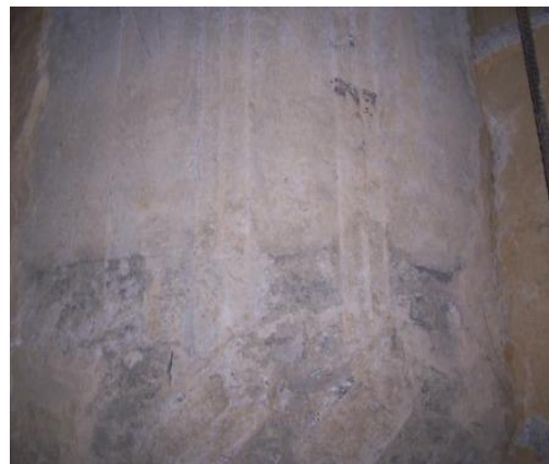
Figure 35: Casing impression marks in N3P9
