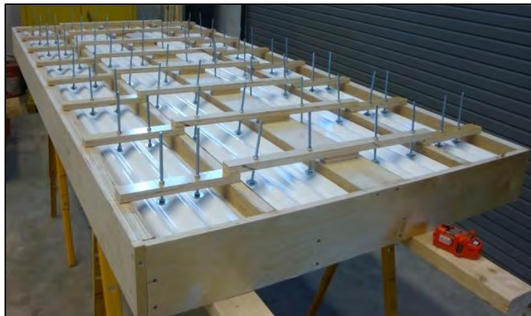
Figure 31: Round corrugated rubber form trough
