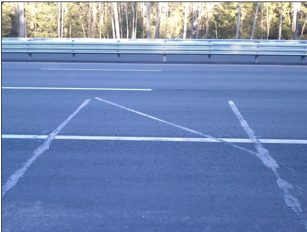
Figure 35: The completed array of axle-sensor strips approximately two weeks after installation.
