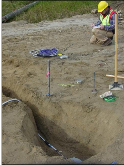
Figure 28: Installation of pressure cell 093461.
