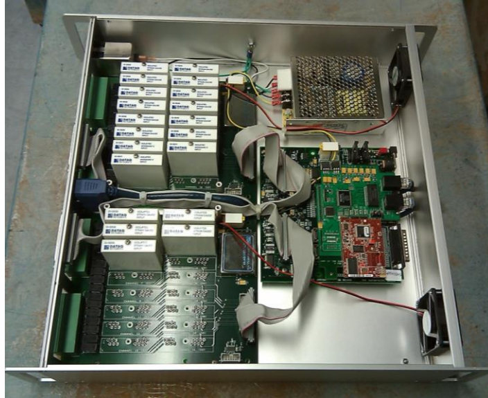
Figure 20: DATAQ DI-785 with signal conditioners installed.
