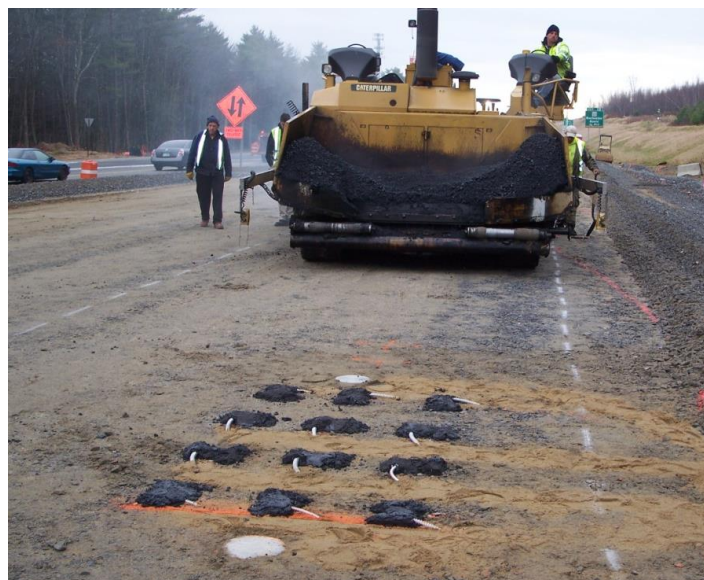
Figure 31: Strain gage array during base course placement.
