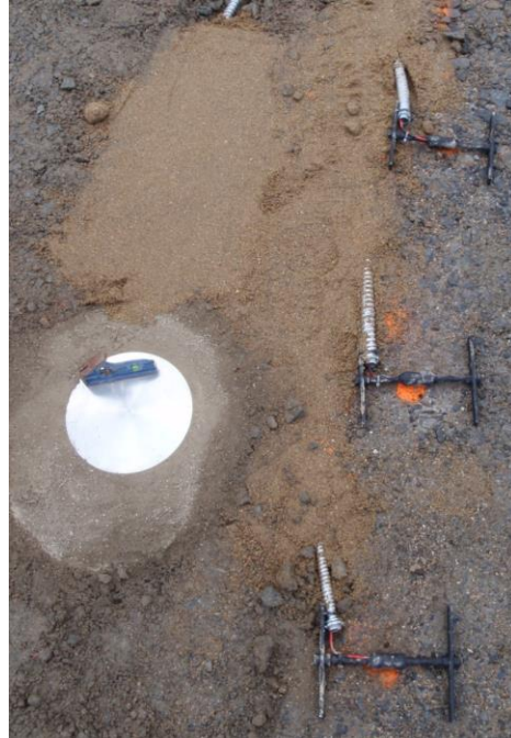
Figure 30: Pressure cell and strain gages prior to paving.
