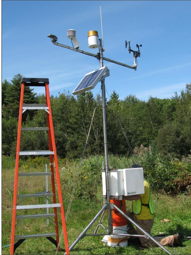
Figure 15: The weather station during the final phase of installation at the site.
