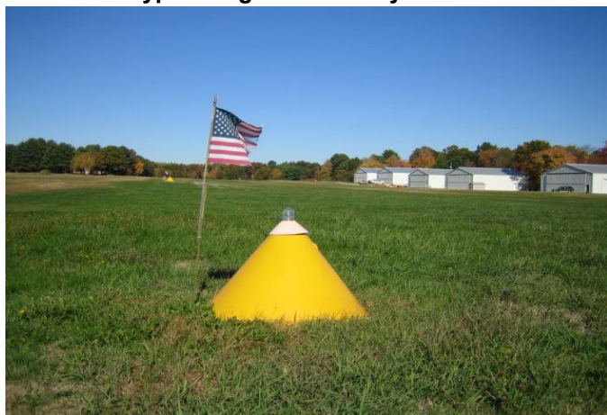
Exhibit 1-3 Typical Lighted Runway Marker
