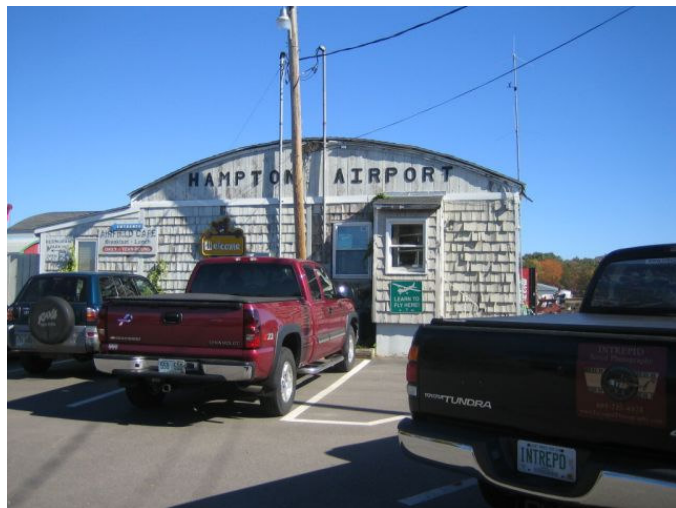
Exhibit 1-2 Original Hangar Building
