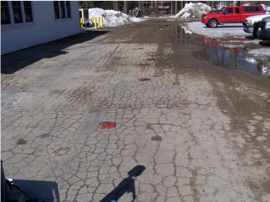
Figure 6: Wentworth Shed looking away from the gas pumps
