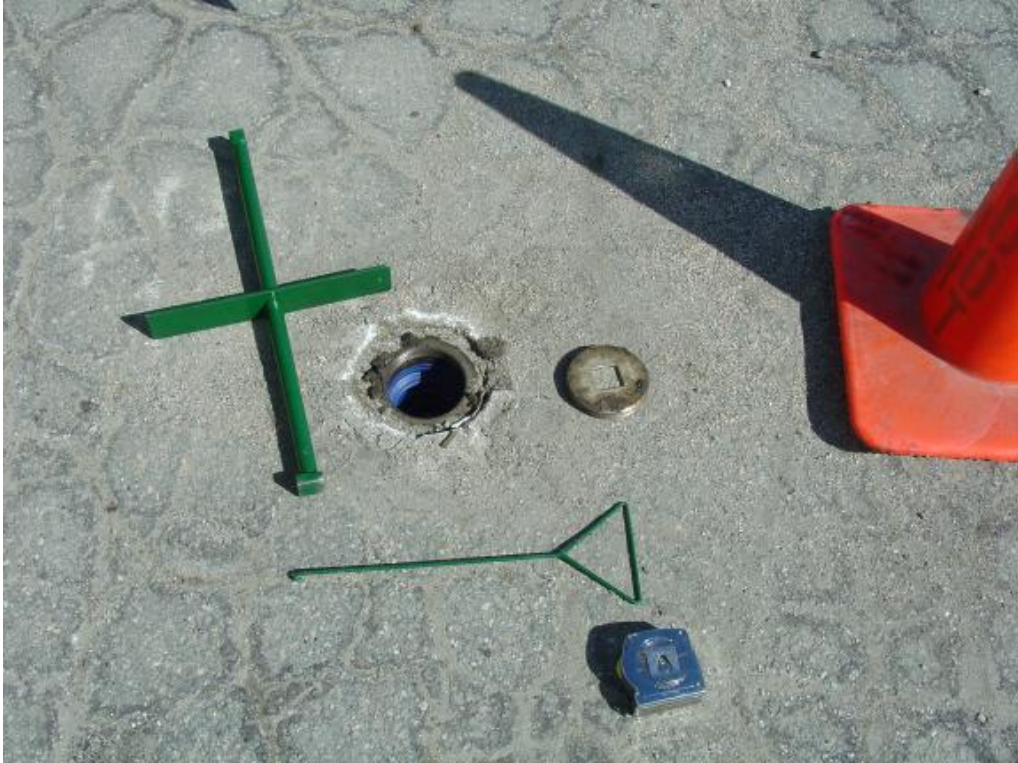
Figure 10: Typical frost tube chamber at a site, the interior necks down to be just larger than the frost tube diameter to minimize the air space around the frost tube.
