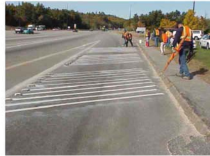
Figure13-b: North view of site
