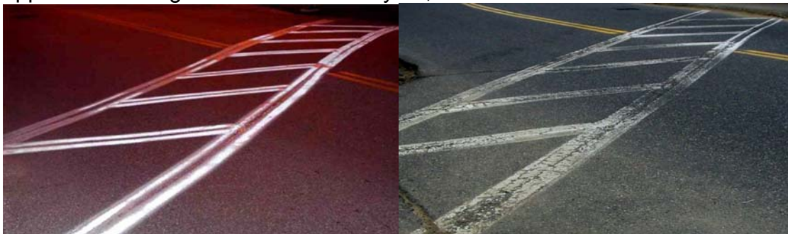
Traffic paint at the Durham test site. Left on August 2002. Right on May 8 th , 2003.
