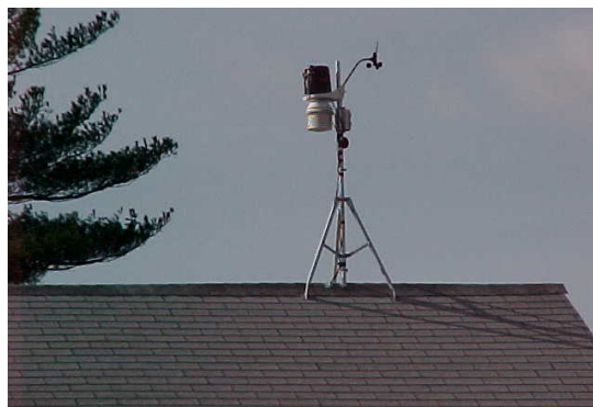
Figure 3: Weather Station at Bristol Maintenance Shed
