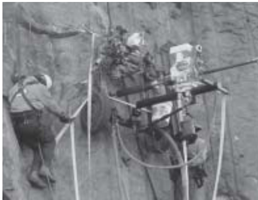
Overcoring to exhume rock reinforcement.
