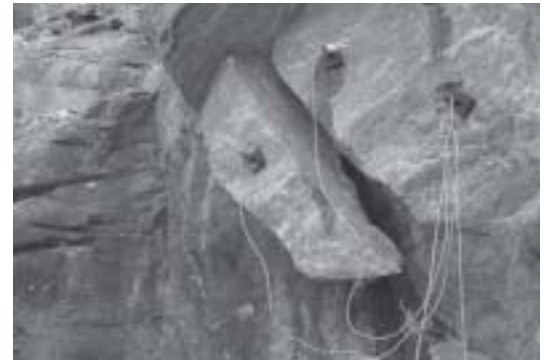
Rock bolts wired for nondestructive testing.
