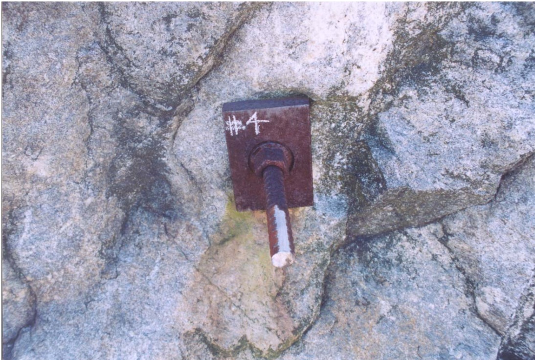
Figure 9. Typical Rock Bolt End Prepared for Testing
