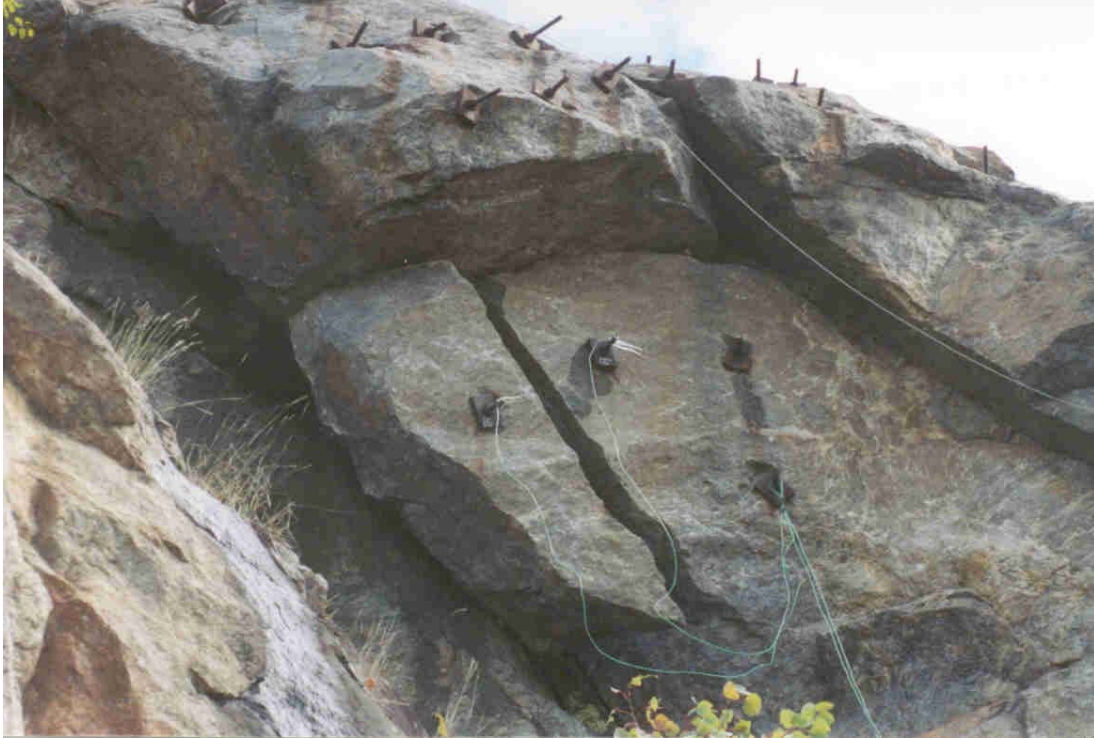
Figure 10. Rock Bolts Wired for Electrochemical Testing
