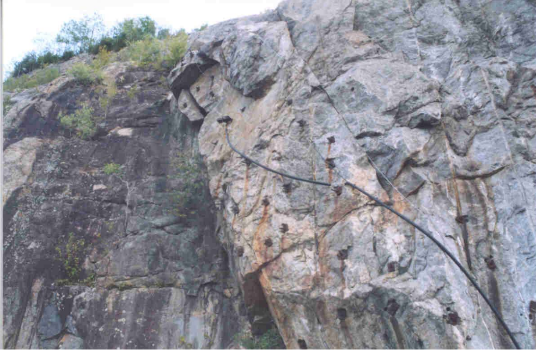
Figure 19. Rockmass Character Near Sta. 1775+25
