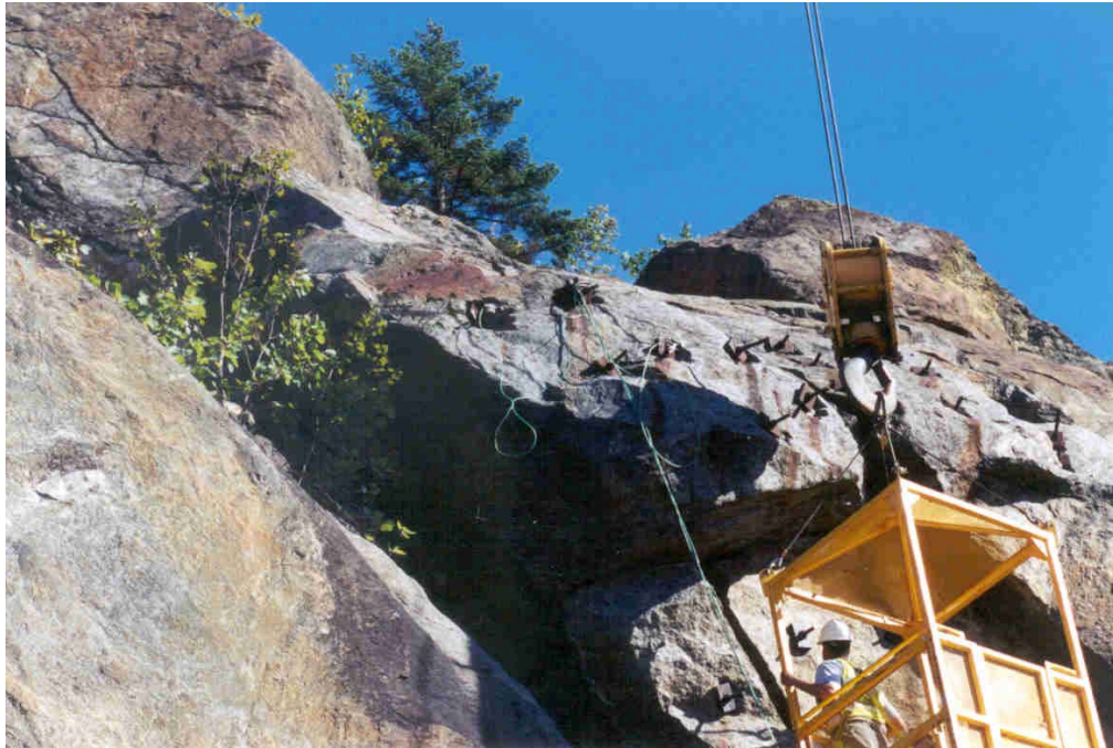
Photograph 13 – Half-cell location for Bolts 17 and 18. Half-cell was placed in a small crack approximately 10 feet to the right of Bolt 18.
