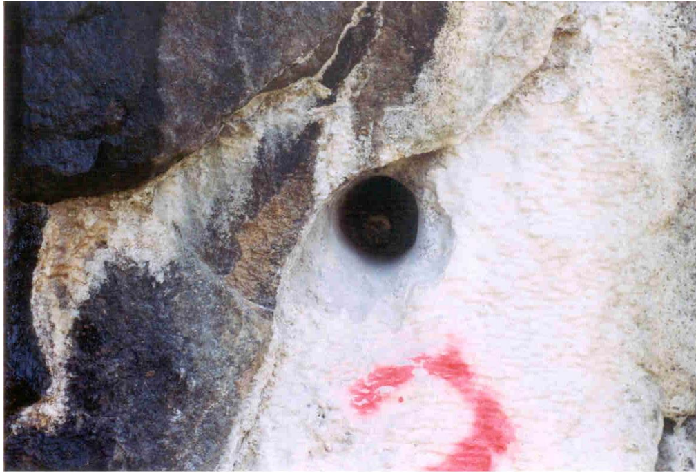
Photograph 3 – Exposed end of Tendon 2-2 after chipping
