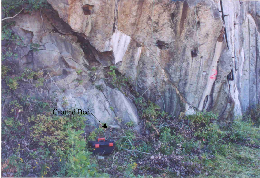
Figure 12. Photo of Ground Bed for Polarization Test
