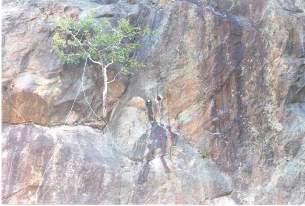
Photograph 1 – Half-cell location for Tendons 1-3 and 1-4.
