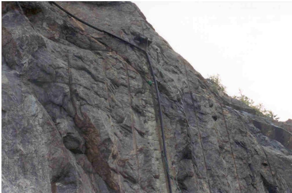
Photograph 6 – Half cell location for Tendons 5-3 and 5-4. Half-cell is placed beneath the black cable conduit approximately three-quarters of the way up the vertical section located in the center of the photograph.
