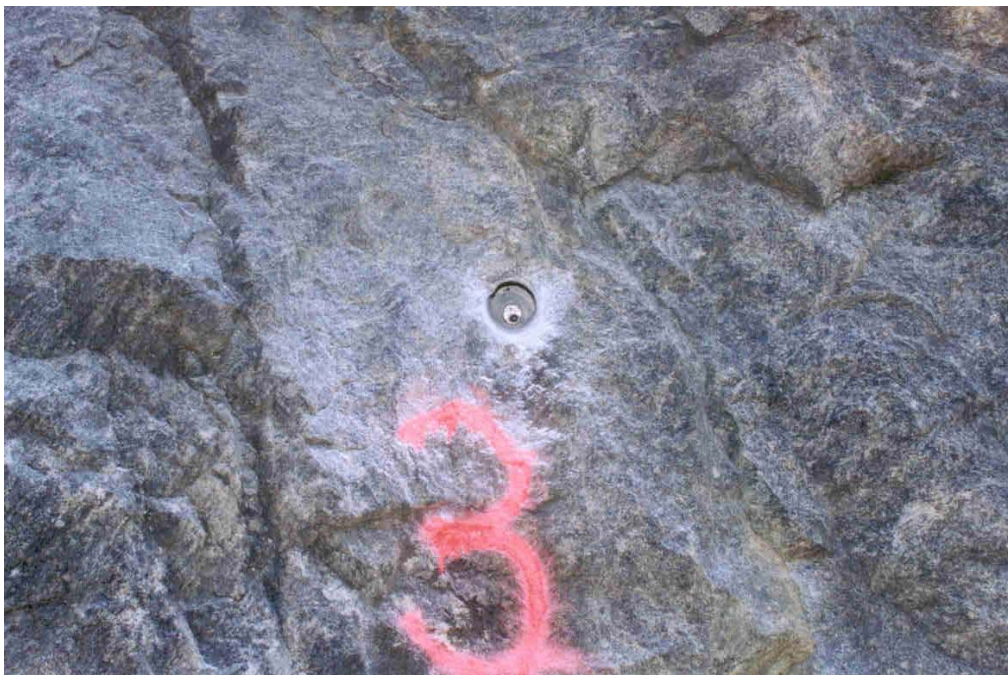
Photograph 3 – Exposed end of Tendon 2-2 after chipping
