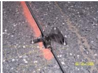
Installation bracket attached to micro nozzle.
