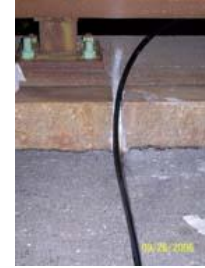
Lateral pavement and curb cuts make way for supply tubing from the median side bridge rail.
