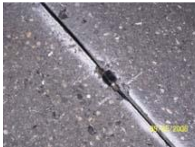
Micro nozzle and tubing laid into pavement groove.
