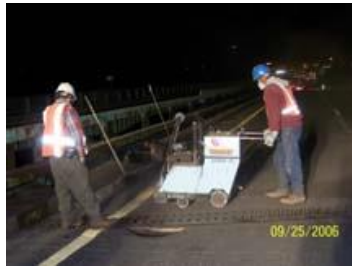
Lateral pavement and curb cuts make way for supply tubing from the median side bridge rail.
