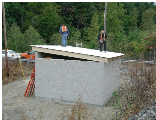
Removable pump house roof system allows for easy storage tank replacement.
