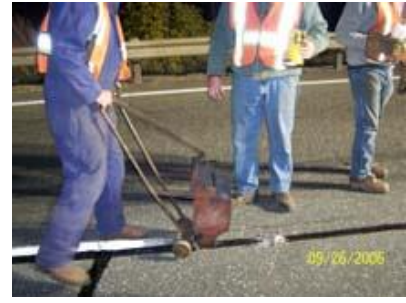
Crack sealant being placed over backer rod and supply tubing.
