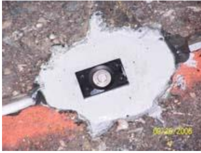
Completed nozzle installation, held in place by epoxy product.
