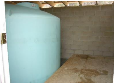
Pump house storage tank and deck.
