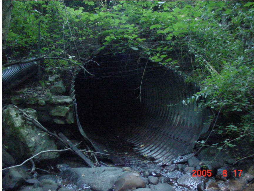
Figure 11: 1.5 meter metal pipe buried beneath 18 meters of roadway fill.
