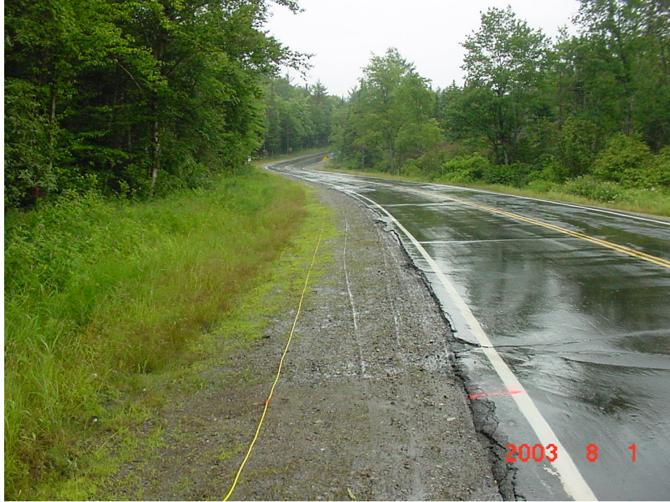
Figure 16: Resistivity line set up along the southern side of the roadway.
