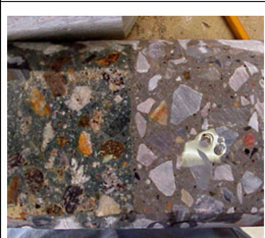
Figure A-10 - Overpour on left, PCP on right prior to failure
