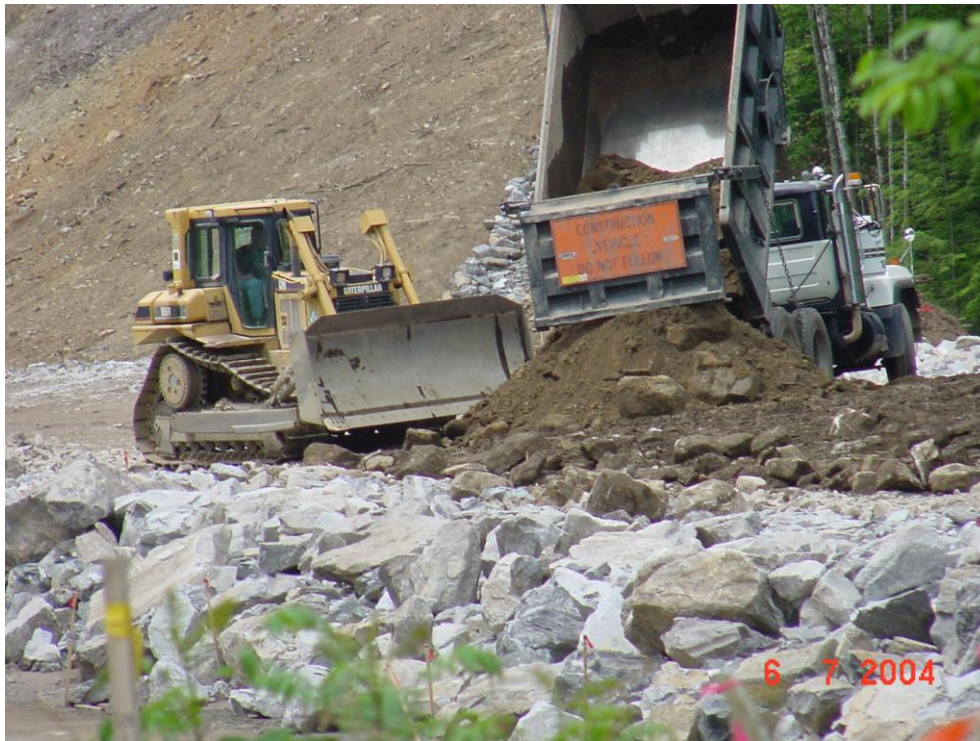
Figure 9 - Bulldozer on rock fill
