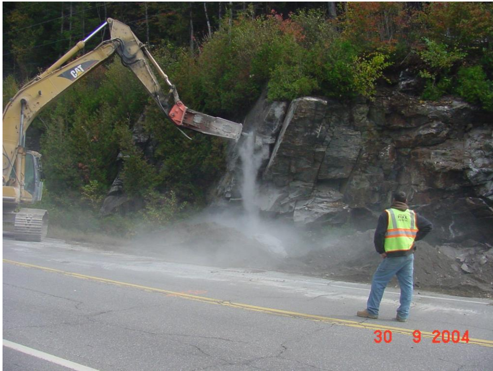
Figure 7 - Hoe-ram breaking up rock
