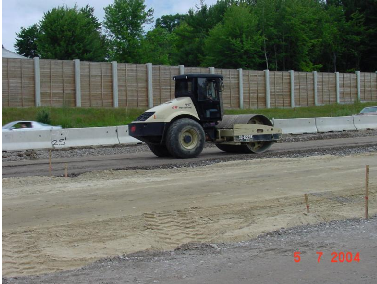
Figure 4 - Vibratory roller compacting base course material
