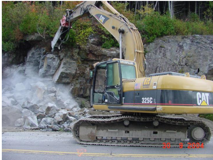
Figure 14 - Track mounted excavator on pavement
